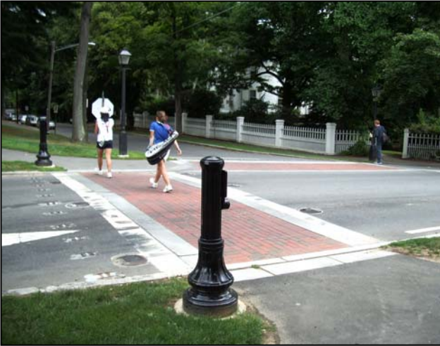
Raised pedestrian walkways (Speed Tables) near Amherst College
