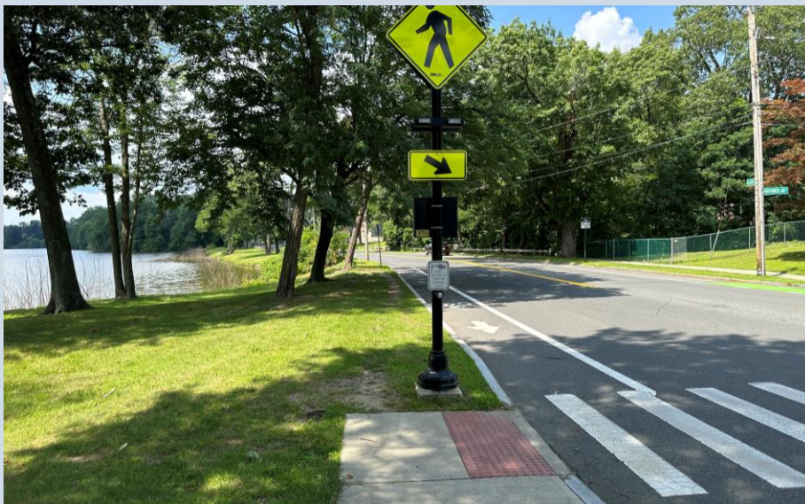
The bicycle lane, sidewalk, and crosswalk added during the recent roadway improvements on Alden Street. The dirt footpath beyond the crosswalk indicates demand for a continuation of the existing sidewalk on this side of the street.
