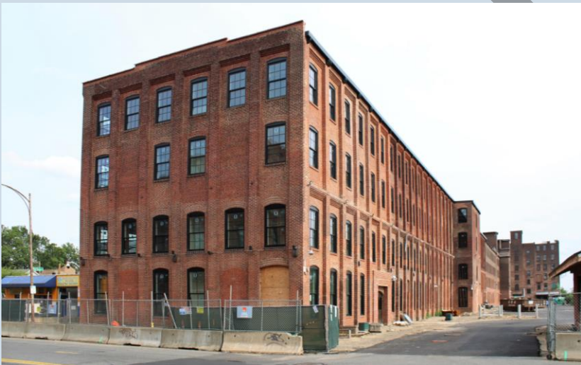
The former Knox Automobile factory, now undergoing conversion into apartments
