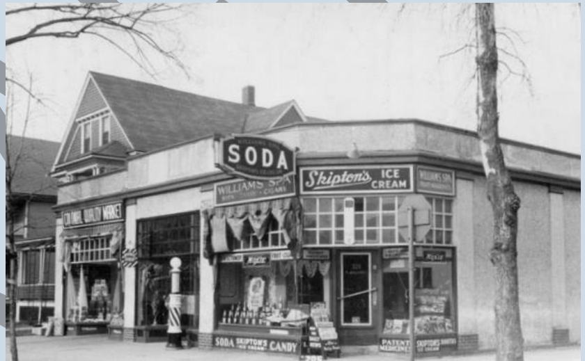
A neighborhood market at the corner of Wilbraham Road and Colonial Avenue, around 1938-1939. Springfield Preservation Trust.
