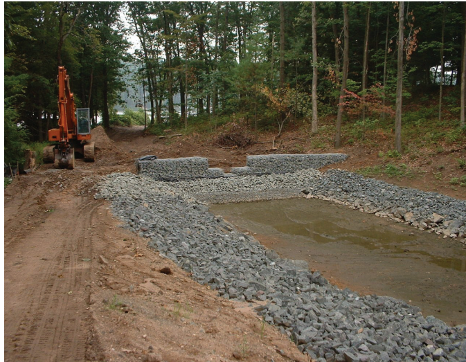
Congamond Lakes Restoration Project, Southwick
