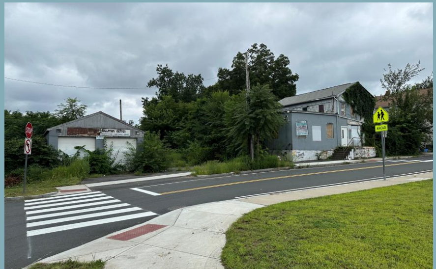
Vacant buildings at the corner of Central and Rifle Streets.
