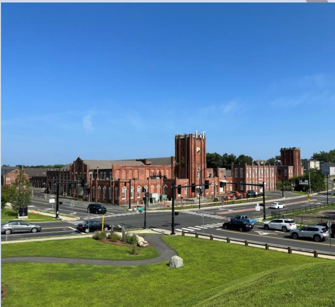
The Armory Watershops facility, seen looking across Allen Street from Ruth Eliabeth Park
