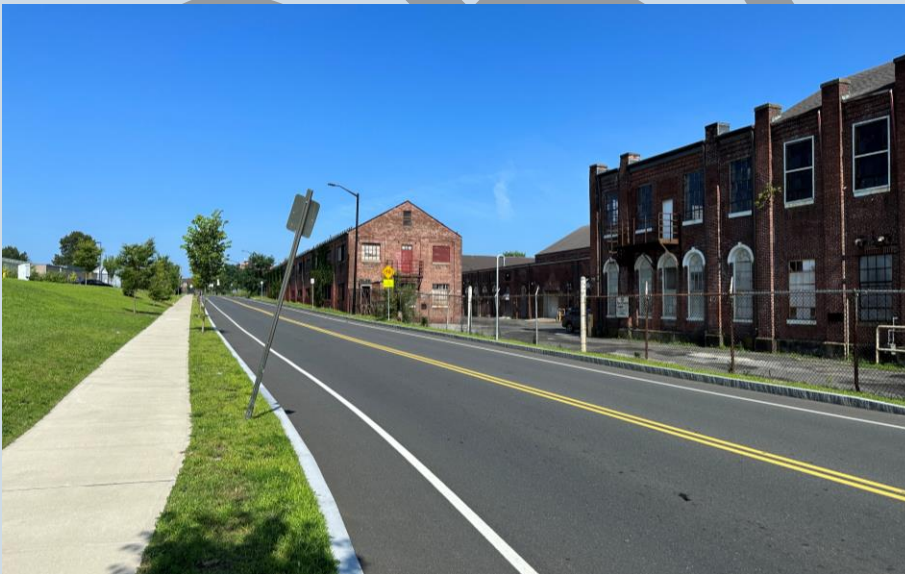
Roadway improvements on Hickory Street, with the Armory Watershops on the right
