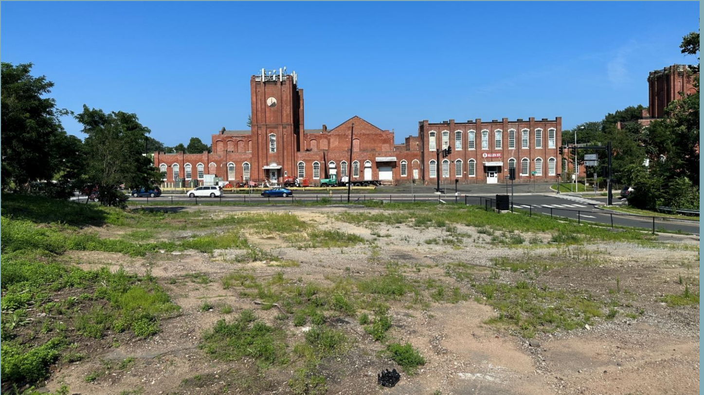
Vacant city-owned land to the east of the One Stop Plaza, with the Armory Watershops in the distance.
