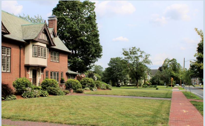
A scene in the Maple Hill Historic District, looking south from near the corner of Maple and Pine Streets.
