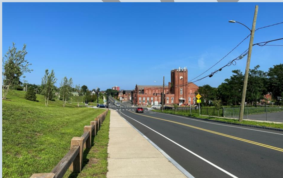
Roadway and sidewalk improvements on Hickory Street. This had previously been a narrow one-way road with no sidewalks.
