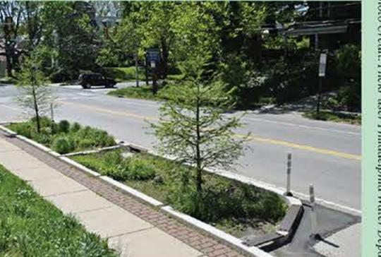
Street edges provide opportunities to receive and manage storm flow from roadways. These facilities, typically in the municipal right-of-way, can also be designed to make streets safer and more comfortable for pedestrians and cyclists by providing shade and separation from motor vehicles, and by "calming" fast-moving vehicular traffic.
