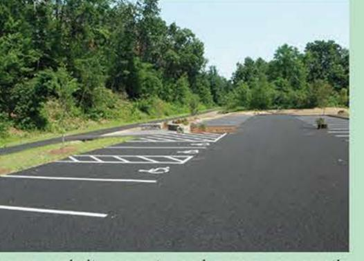
Porous asphalt, concrete, and pavers can greatly reduce stormwater impacts without sacrificing the number of spaces in a parking lot. A combination of traditional asphalt in drive lanes and porous asphalt in parking stalls allows heavy vehicles, such as school buses or delivery trucks, to drive without risk of compacting the porous material.
