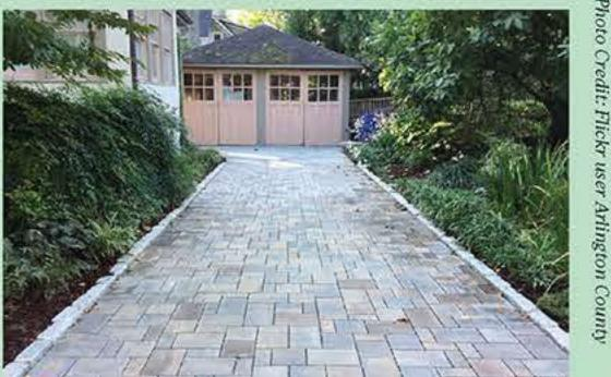
Many residential driveways need not be paved with asphalt or concrete. There are many attractive options, such as grass pavers or porous pavers. These alternative materials can also help to prevent pooling of water and ice on driveways during winter months.
