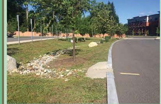
Rain gardens (and bioretention basins) are designed to receive and soak up rainfall. They often include an outlet that allows overflow from larger storms to move into the storm drain system. A vegetated swale looks similar to a rain garden, but is meant to soak up rainfall while also slowly conveying flow from one place to another.
