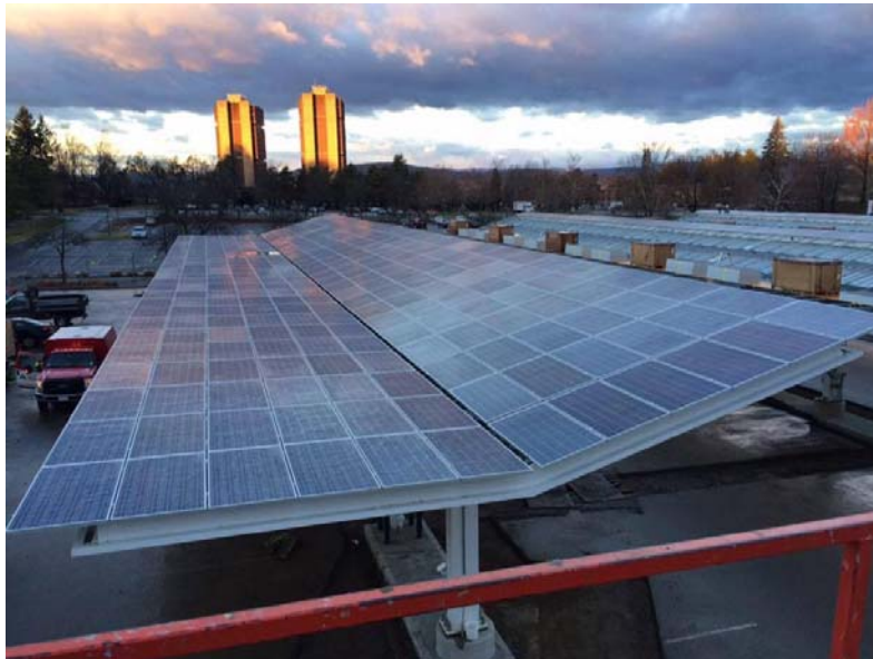
Figure 7: 1,927-kW parking canopy system located on 4.6 acres of parking lot space at UMass Amherst
