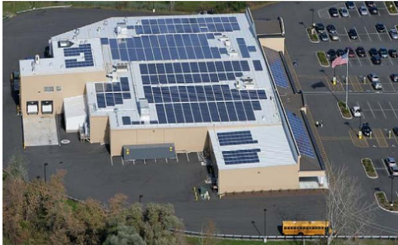
Figure 6: 363-kW rooftop system located on a Big Y grocery store in Lee, MA
