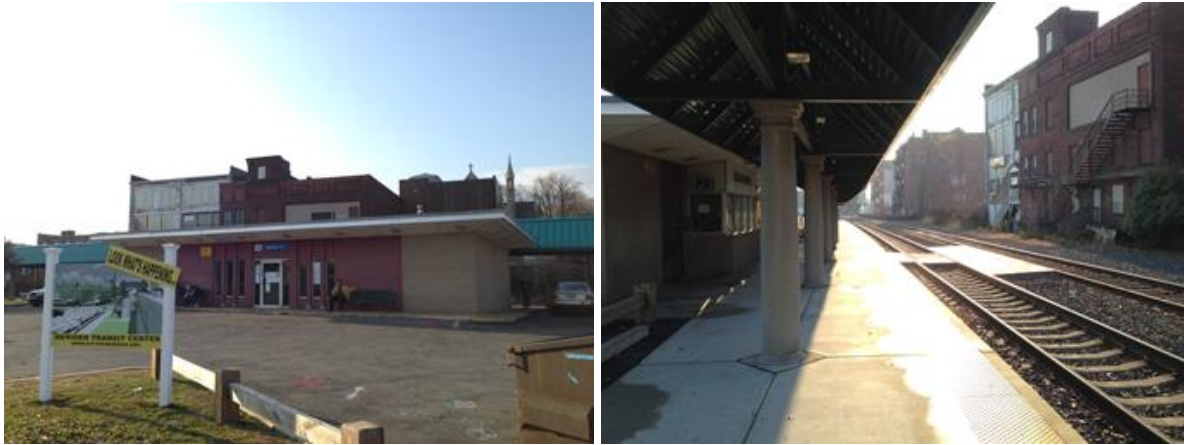
Figures D-31 and D-32. Meriden Station Headhouse, Parking & Platform
