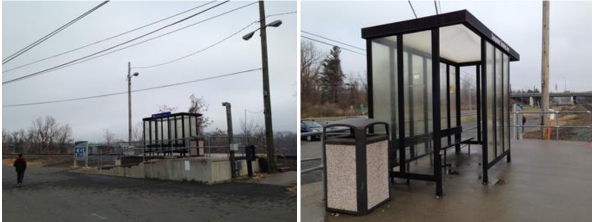
Figures D-20 and D-21. Windsor Locks Station Platform
