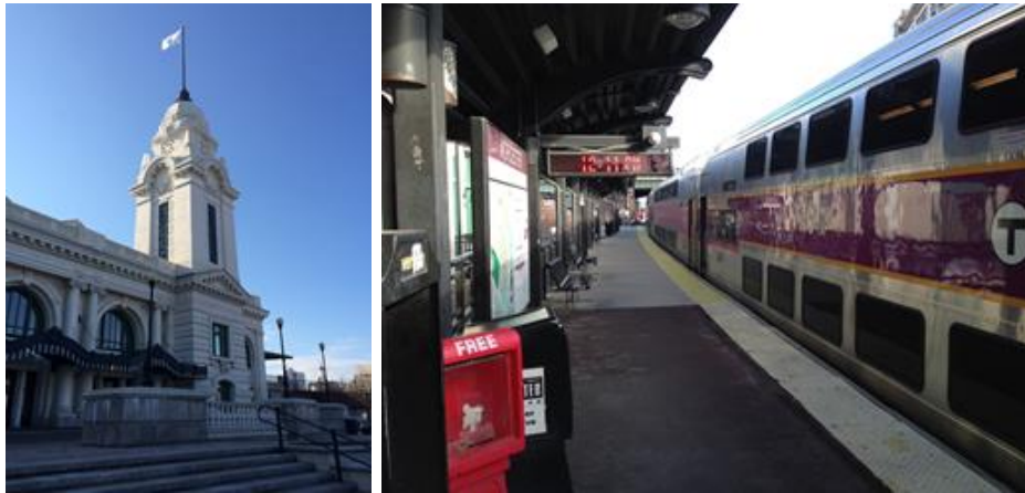
Figures D-9 and D-10. Worcester Union Station Headhouse and Platform
