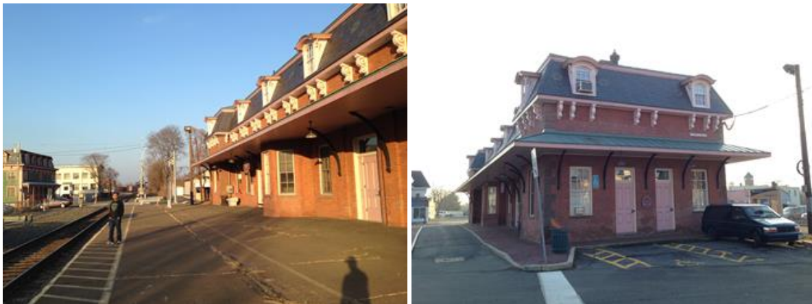
Figures D-34 and D-35. Wallingford Station Headhouse, Parking, and Platform
