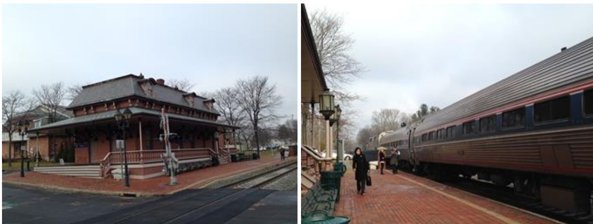
Figures D-23 and D-24. Windsor Station Headhouse and Platform
