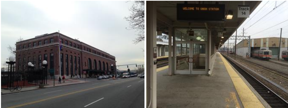
Figures D-36 and D-37. New Haven Union Station Headhouse and Platform
