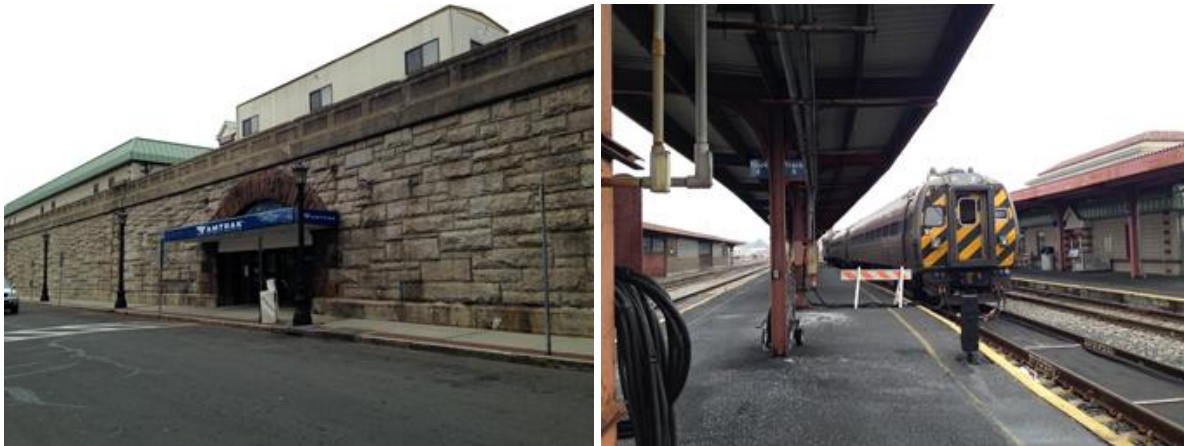
Figures D-15 and D-16. Existing Springfield Union Station Headhouse and Platform Area
