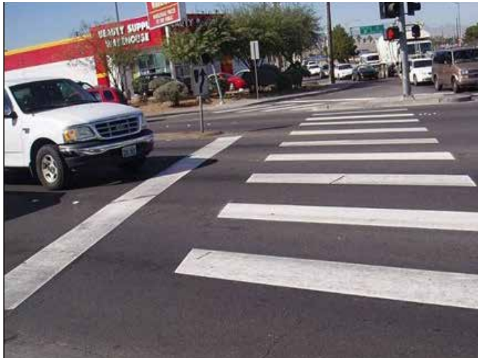
Crosswalk and stop line Source: http://safety.fhwa.dot.gov/ped_bike/tools_solve/ped_scdproj/sys_impact_rpt/images/fig16.jpg
