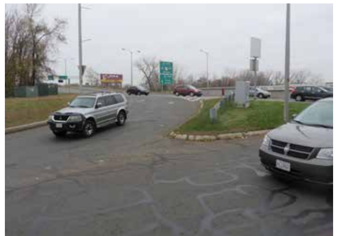
A right-turn slip lane without any crosswalks currently enables westbound traffic on Route 20 to turn north onto Plainfield Street at high speeds without slowing down, creating a risk of vehicular and pedestrian accidents.
