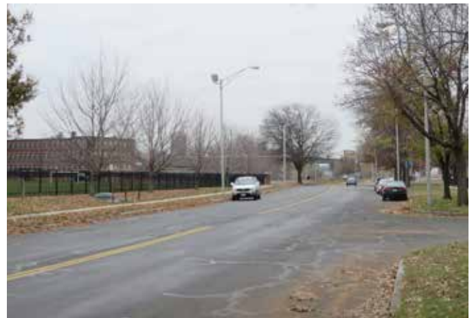
Wide travel lanes and a lack of crosswalks currently contribute to high traffic speeds and unsafe pedestrian conditions on Plainfield Street.
