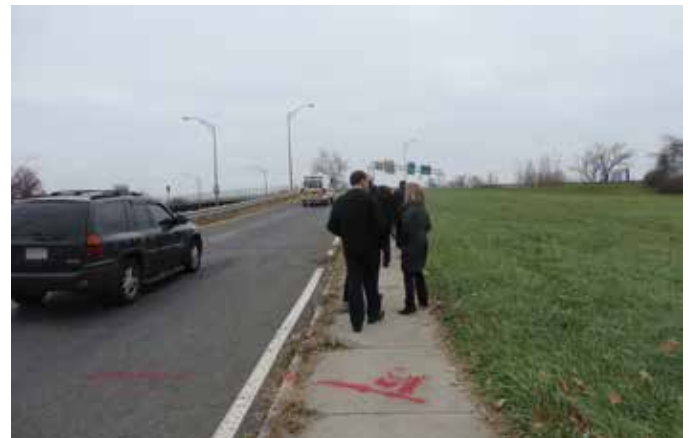
No buffer exists between pedestrians and high-speed traffic along the Birnie Avenue ramp on the approach to Route 20/Plainfield Street.
