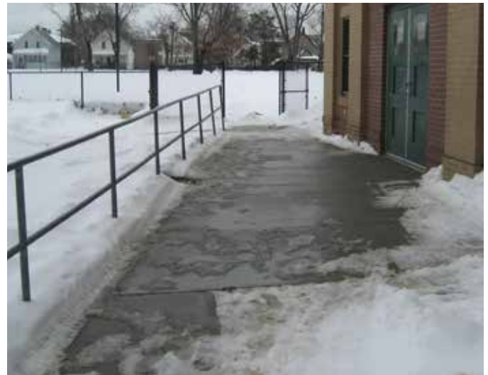
School walkways were not cleared near entrance doors along the northern side of the school
