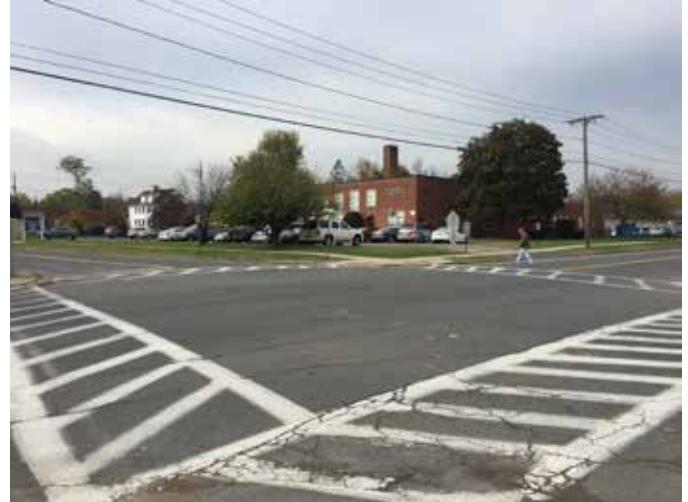
Well-marked, ladder crosswalks are at both major intersections near Memorial Elementary School.
