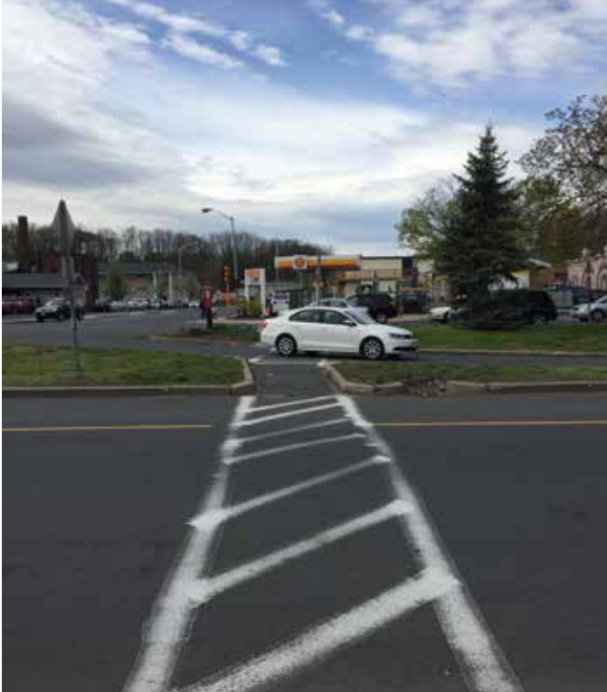
View of the Elm Street crosswalk looking west toward Westfield Street
