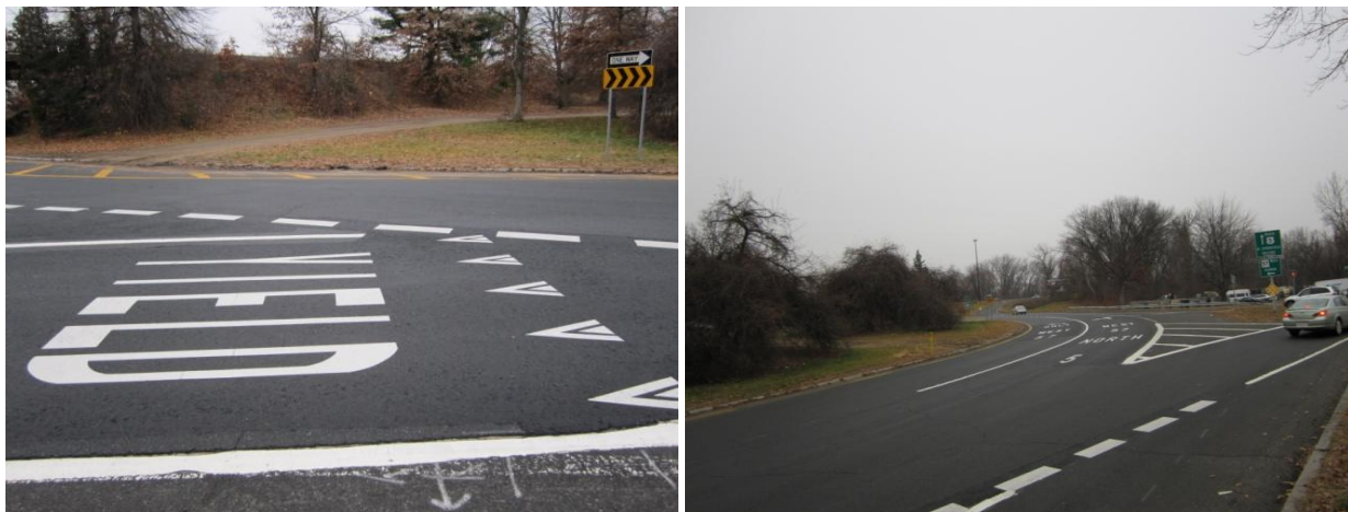
The Agawam Route 5 / Route 57 Rotary Views from South End Bridge Approach Source: PVPC
