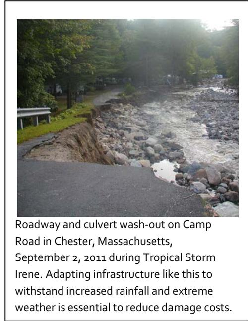
Roadway and culvert wash-out on Camp Road in Chester, Massachusetts, September 2, 2011 during Tropical Storm Irene. Adapting infrastructure like this to withstand increased rainfall and extreme weather is essential to reduce damage costs.
