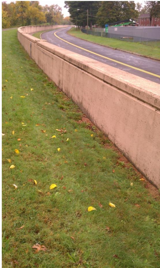
The levee protecting Springfield's North End neighborhood has shifted over time, creating a slope that causes water to pool next to it. This is causing damage to the levee foundations and will eventually require costly improvements. Source: PVPC
