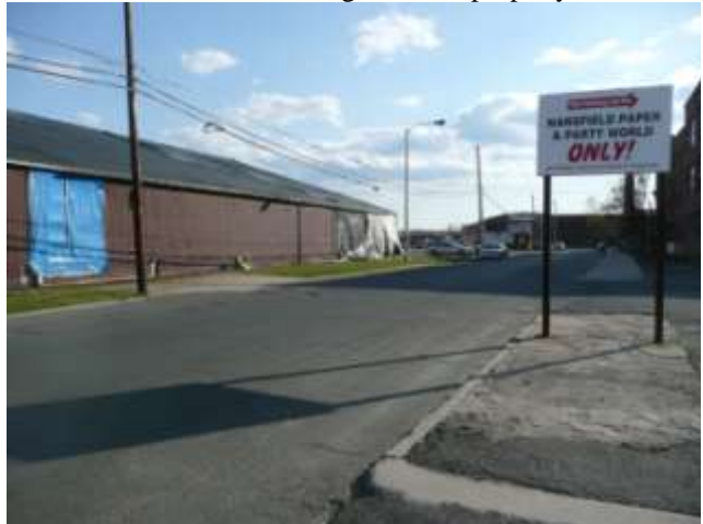
Cold Spring Ave view to southwest
