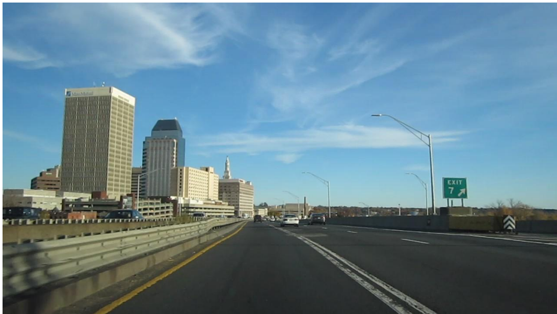
Figure 63 - No Passing Zone in the Left Lane from I-291 to I-91 Southbound Near Exit 7.
