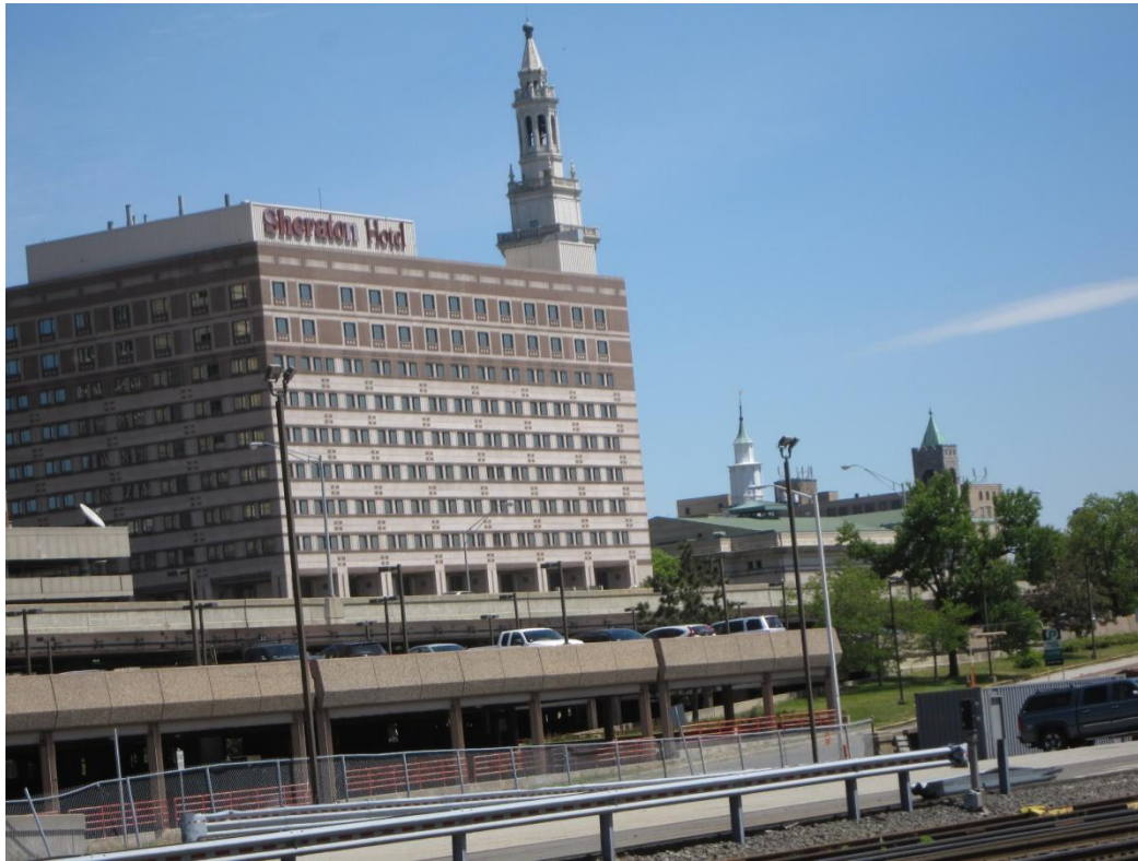
Figure 56 - I-91 South Parking Garage, Springfield.
