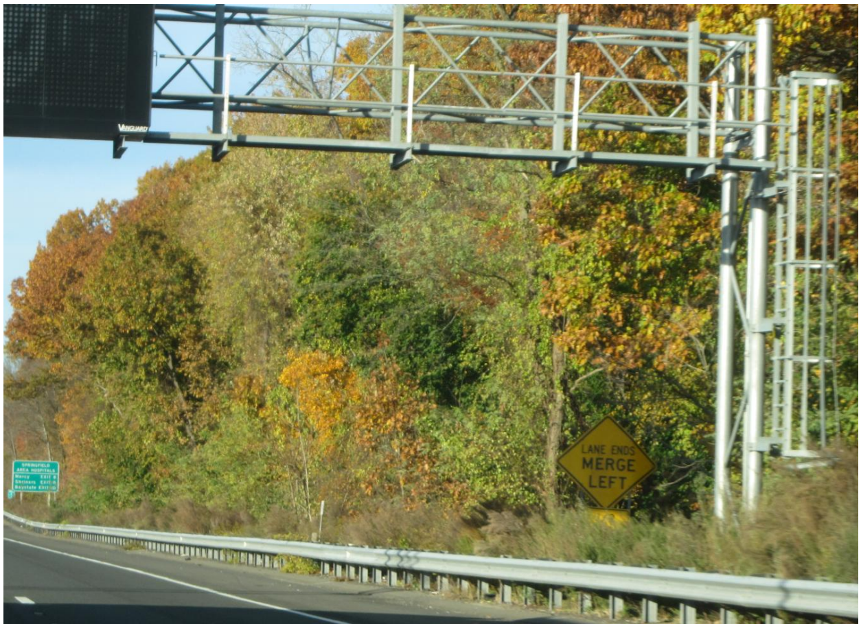
Figure 77 - "Lane Ends Merge Left" Warning Sign Hidden by Signage Structure Over I-91 Northbound.
