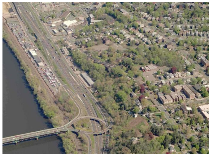
Figure 3 - South End Bridge Arial View.
