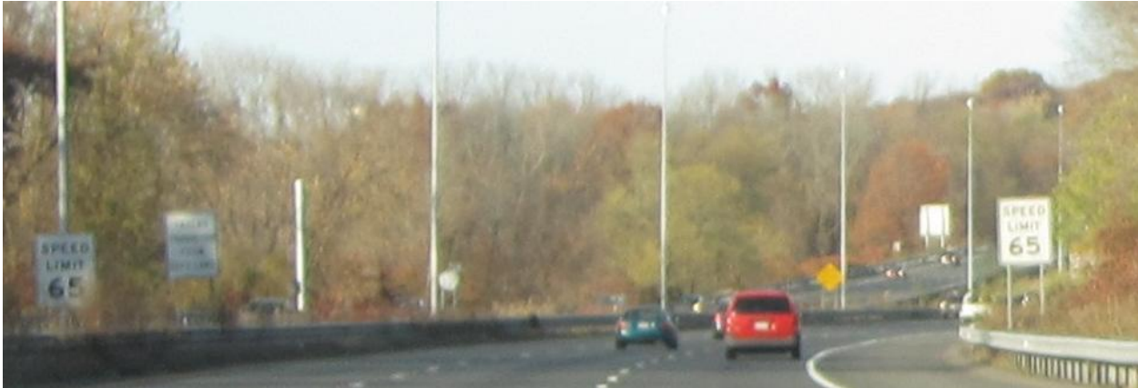
Figure 72 - Speed Limit Sign Set at Low Height and Obscured by Vegetation.
