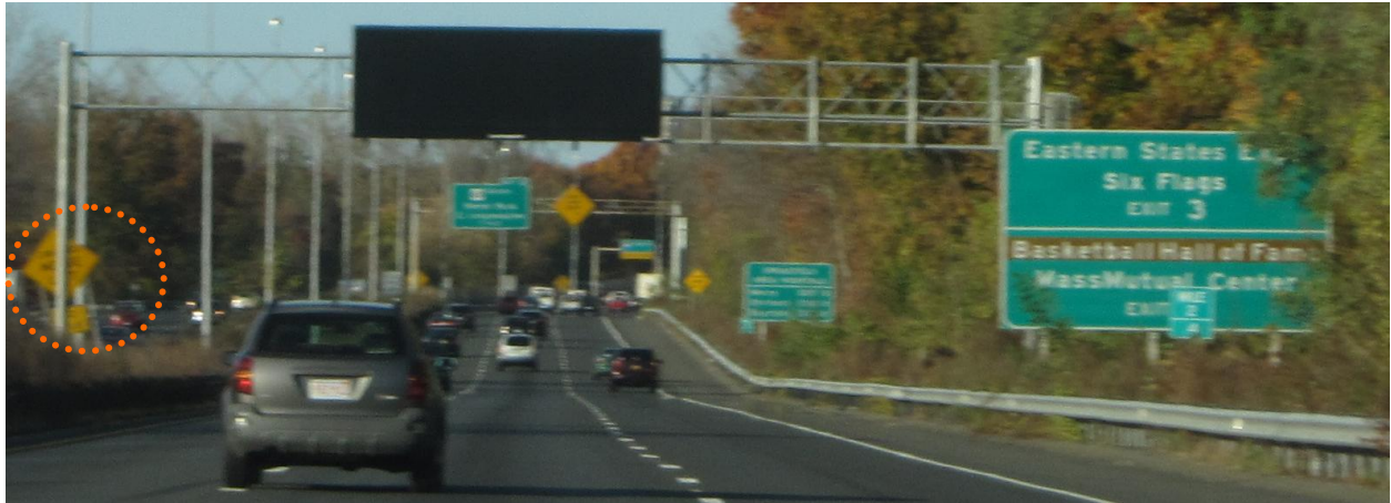
Figure 77 - "Lane Ends Merge Left" Warning Sign Hidden by Signage Structure Over I-91 Northbound.
