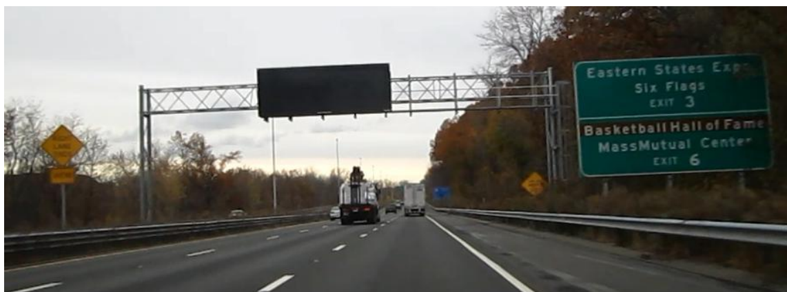
Figure 102 - Variable Message Board Over I-91 Northbound Near Exit 3.
