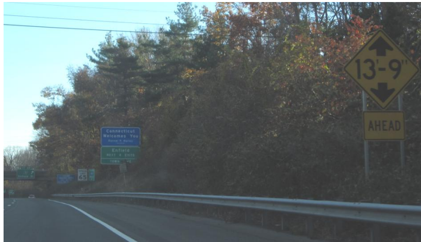
Figure 70 - Bridge Height Warning Sign Before State Line Obscured by Vegetation.
