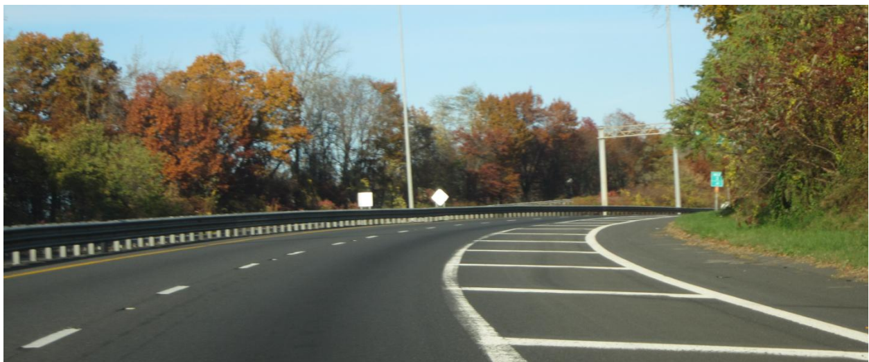
Figure 82 - Wide Roadway Shoulder After Lane Drop on I-91 Northbound Before Exit 2.
