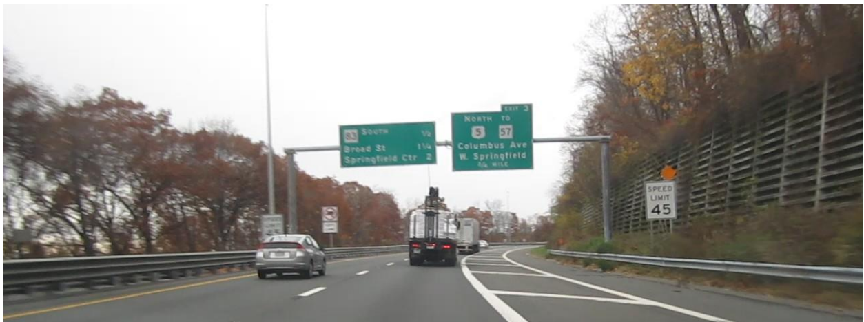
Figure 82 - Wide Roadway Shoulder After Lane Drop on I-91 Northbound Before Exit 2.
