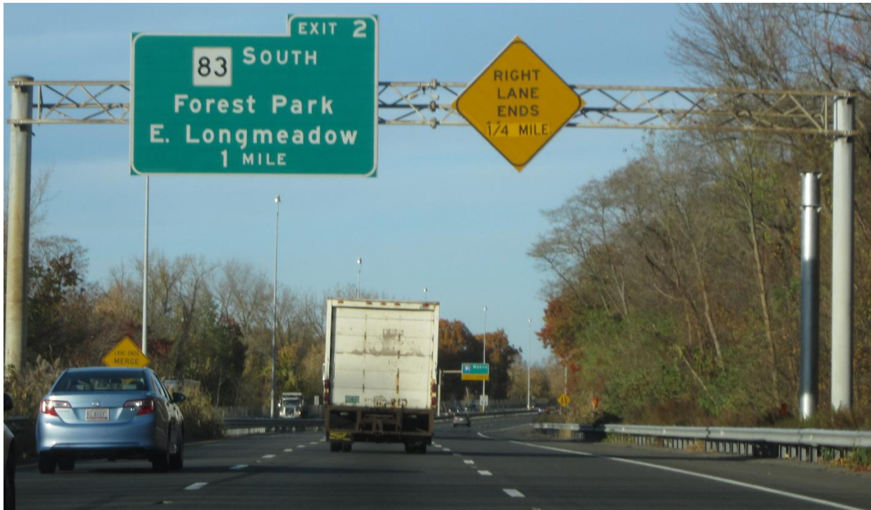
Figure 79 - Lane Drop Taper on I-91 Northbound Before Exit 2.
