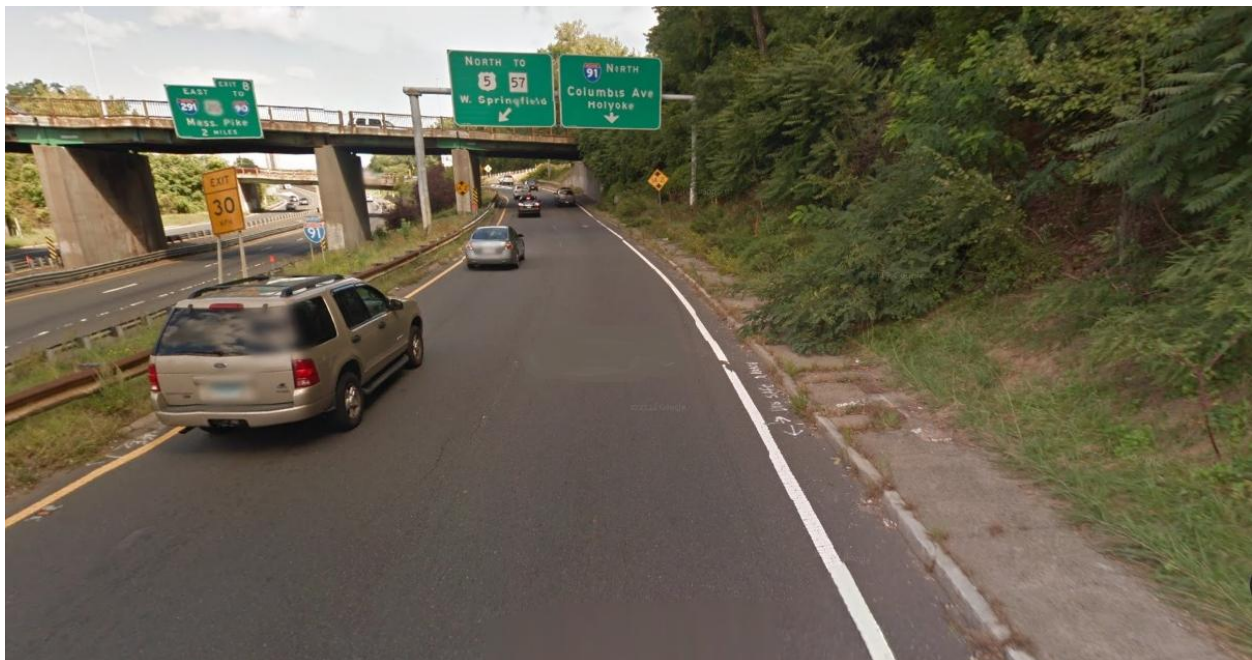
Figure 102 - I-91 Northbound Exit 3 Ramp is Narrow and Lacks Warning Sign for Upcoming Weave.
