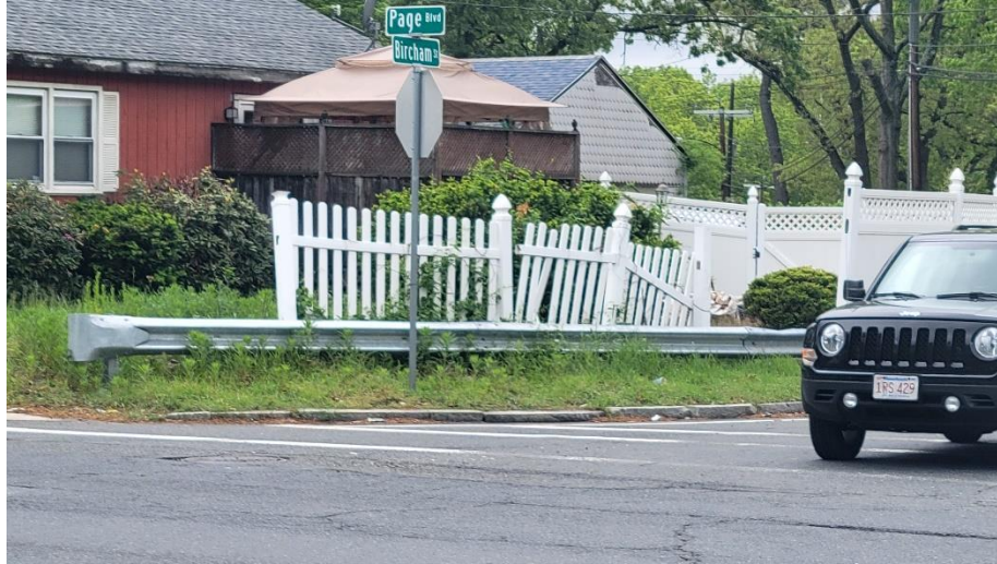
Figure 2: Guard Rail and Damaged Fence along Northwest corner of the Intersection
