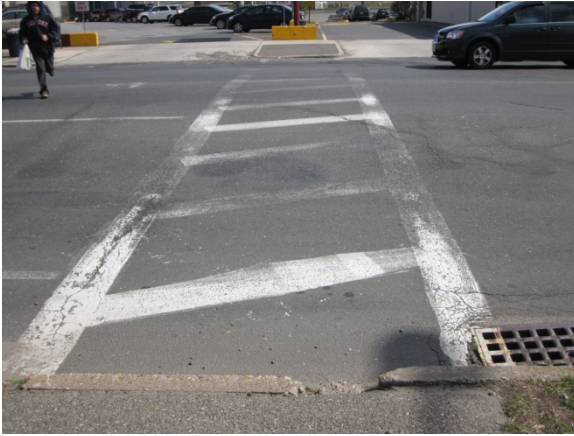
Non ADA compliant pedestrian crossing
