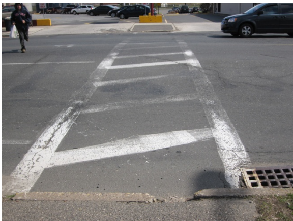
Non ADA compliant pedestrian crossing
