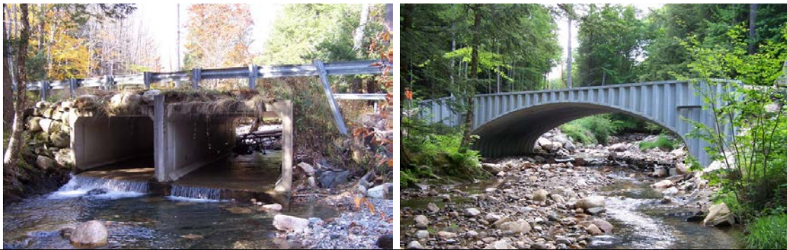
Dingle Road crossing of Bronson Brook, Worthington, before and after. (Credit: Carrie Banks)
