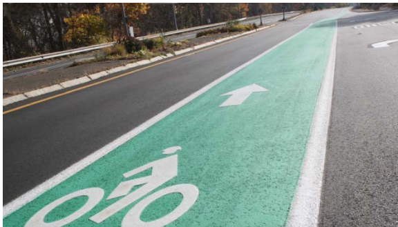
New bike lane on Route 5 in Holyoke
