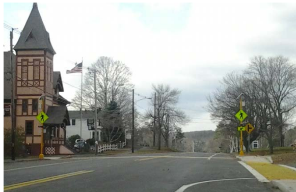
New pedestrian crossing in Brimfield
