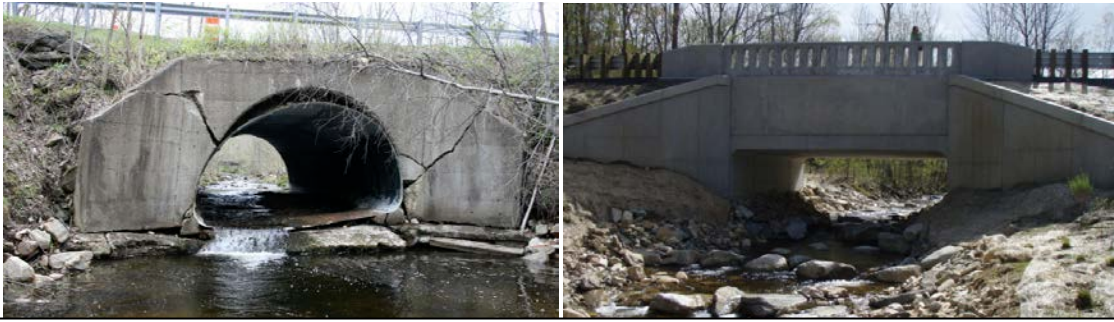
McNearney Road crossing of Shaker Brook, Becket, before and after. (Credit: Carrie Banks)
