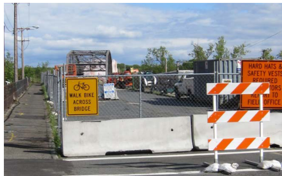
Route 116 Bridge from Holyoke to Chicopee closed for repairs
