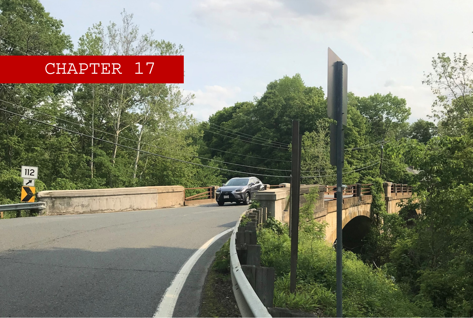
Photo: Route 112 Bridge in Huntington, MA
