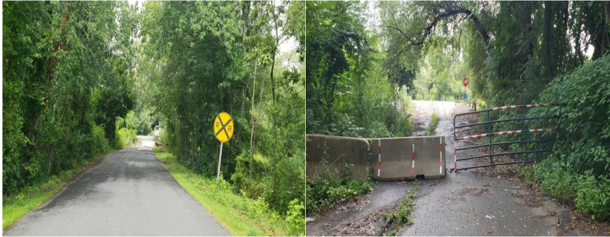
Figure 13: Birnie Road Northbound Approach; Advance Warning Sign and Barriers
