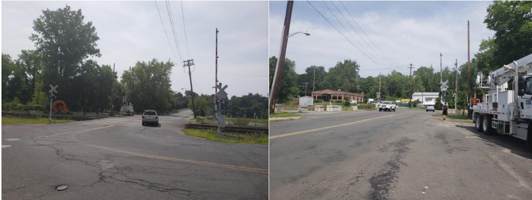
Figure 3: Cross Bucks and Gates along West Springfield side approach (left) and Agawam Side Approach
