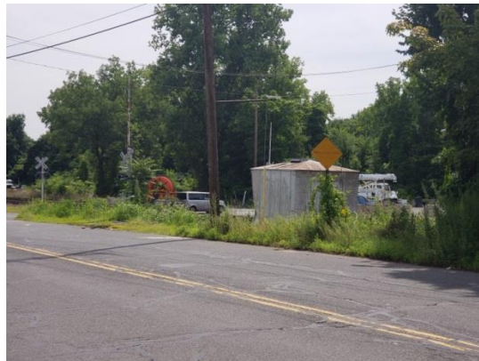
Figure 4: Faded Advance Warning Sign along Front Street
