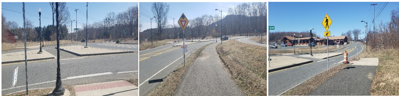
From Left: (i) Northbound approach of the side path depicting the median and faded crosswalk markings, (ii) Eastbound approach of West Bay Road, (iii) Westbound approach of West Bay Road depicting the crosswalk sign
