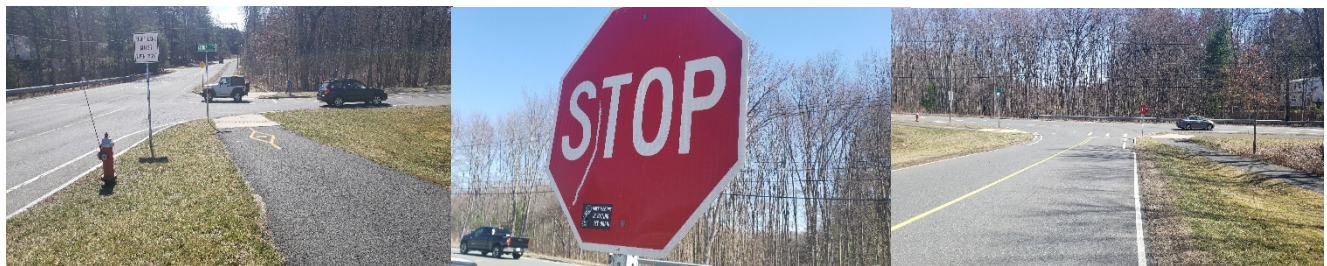
From Left: (i) Southbound approach of the Side Path depicting the location of uninstalled bollard and street name signs, (ii) Vandalized Stop sign at the Kendall Drive approach, (iii) Eastbound approach of Kendall Drive depicting the westbound branch of the SIDE PATH parallel to the road.
