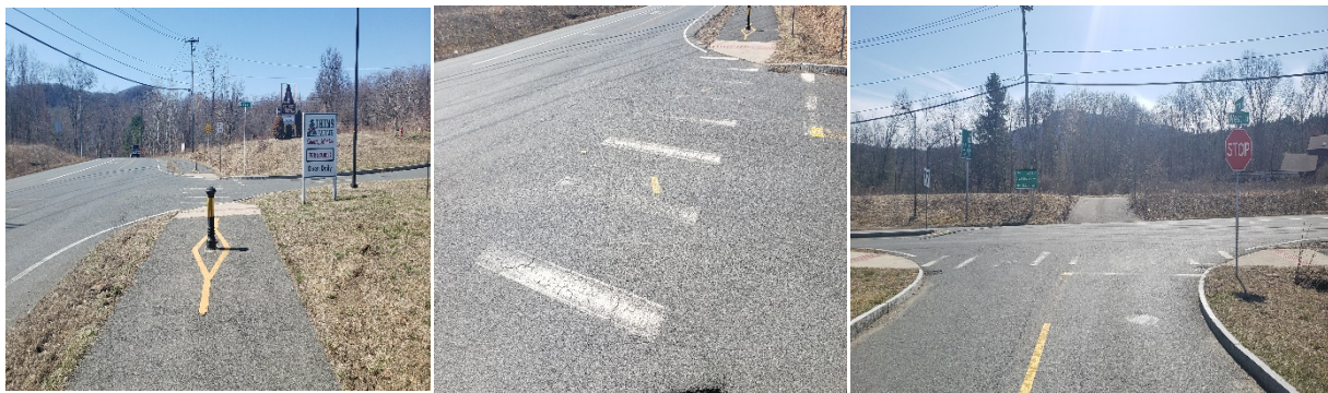
From Left: (i) Southbound approach of the side path with bollard, (ii) Faded crosswalk markings and stop line for Lannon Lane, (iii) Eastbound approach of Lannon Lane and driveway to the east of the intersection with West Street (Route 116)
