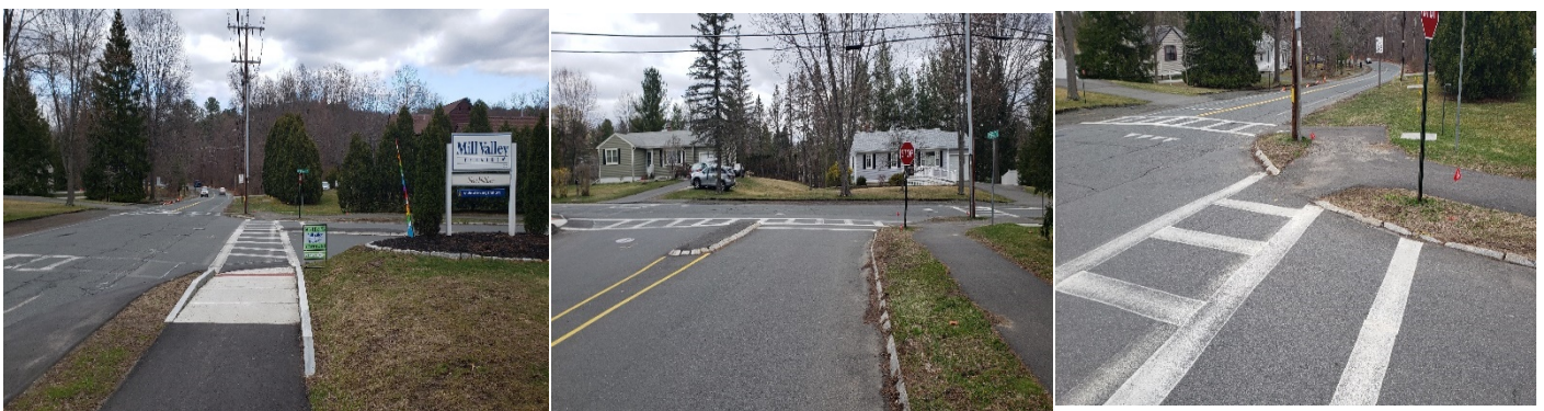
From Left: (i) Eastbound approach of side path with concrete ramp, (ii) Northbound approach of Riverdale Drive with median, (iii) Crosswalk and ramp along westbound approach of the side path
