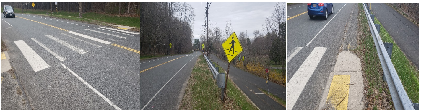
From Left: (i) Crosswalk view from sidewalk along west side of the road, (ii) Southbound approach of North Main Street depicting the damaged sign post, (iii) Ramp along the sidewalk along the west side of North Main Street.
