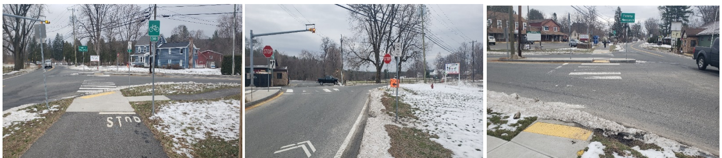
From Left: (i) Westbound approach of the side path depicting the median and faded crosswalk markings, (ii) Southbound approach of Pomeroy Meadow Road, (iii) Eastbound end of sidewalk and faded crosswalk markings
