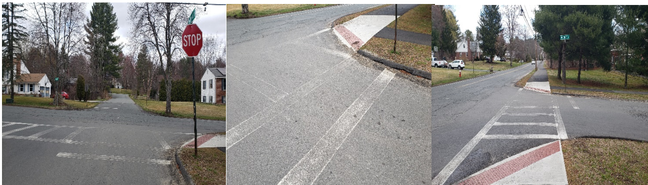
From Left: (i) Northbound approach of Southpoint Drive, (ii) Faded stop line and crosswalk markings, (iii) Eastbound approach of the side path
