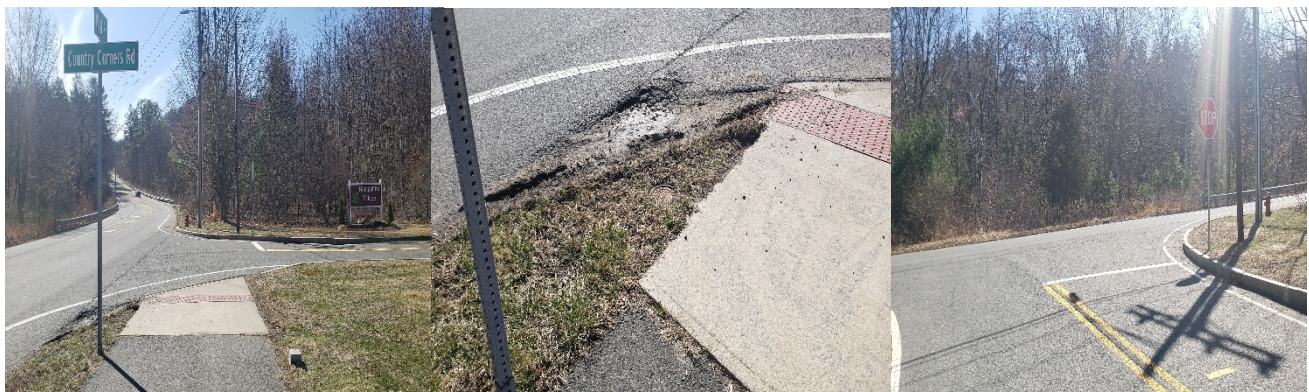
From Left: (i) Southbound approach of the side path, (ii) Northwest corner of the intersection of West Street (Route 116) and Country Corners Road, (iii) Eastbound approach of Country Corners Road
