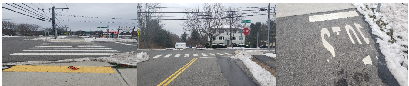
From Left: (i) Westbound approach of the Side Path, (ii) Parc Place approach, (iii) Pavement markings at the eastbound approach of the Side Path
