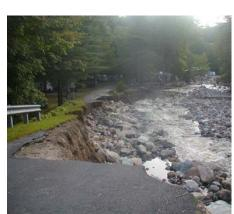
Roadway and culvert wash-out on Camp Road in Chester, Massachusetts, September 2, 2011 during Tropical Storm Irene. Adapting infrastructure like this to withstand increased rainfall and extreme weather is essential to reduce damage costs.
