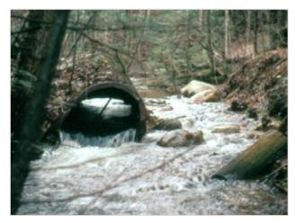
Culverts can fail if stormwater flow exceeds their designed capacity.
