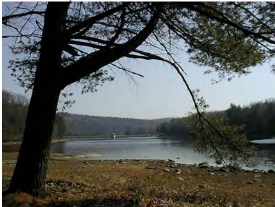
Granville Reservoir and Dam Source: Anne Capra. PVPC
