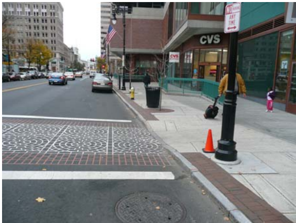
Near the middle of the study area, Town Square, Monarch Place and other large buildings are major trip generators.
