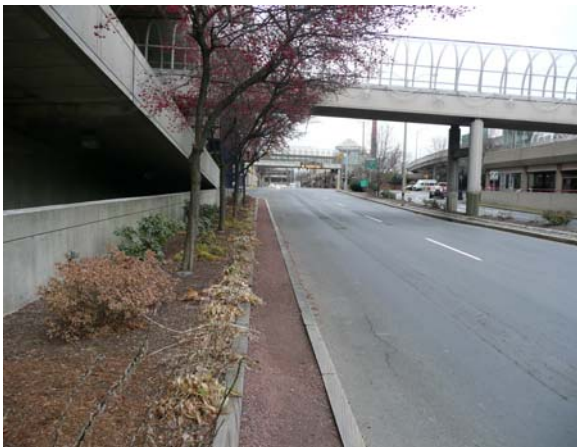
Some sections along East Columbus Avenue have no sidewalk; pedestrians must use this dirt path instead.
