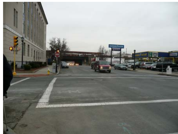
Dwight Street at Taylor Street (State Office Building seen at left). Crosswalks with signals offer pedestrians safety along this portion of the corridor, but there is relatively little street furniture.
