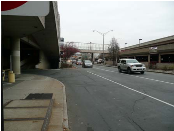
Seen above is the entrance to the Town Square parking ramp, which is the rear of the building. This structure blocks pedestrian egress and passage along the street.
