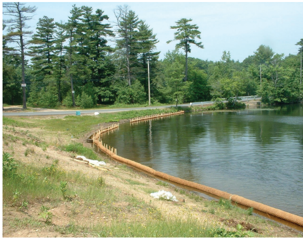
Pequot Pond restoration project, Southampton
