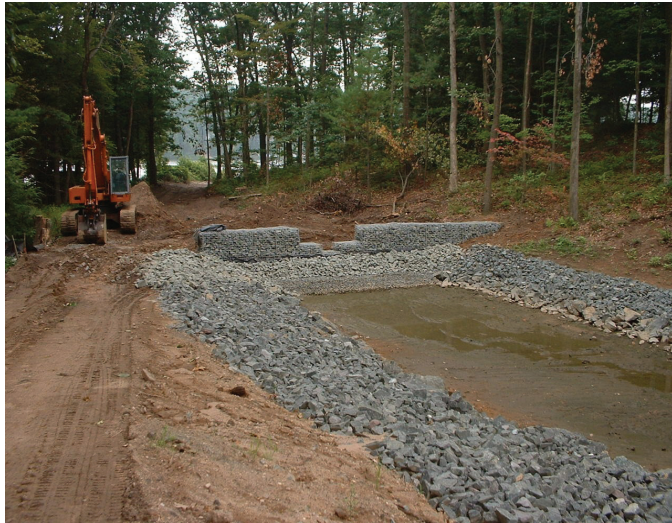
Congamond Lakes Restoration Project, Southwick
