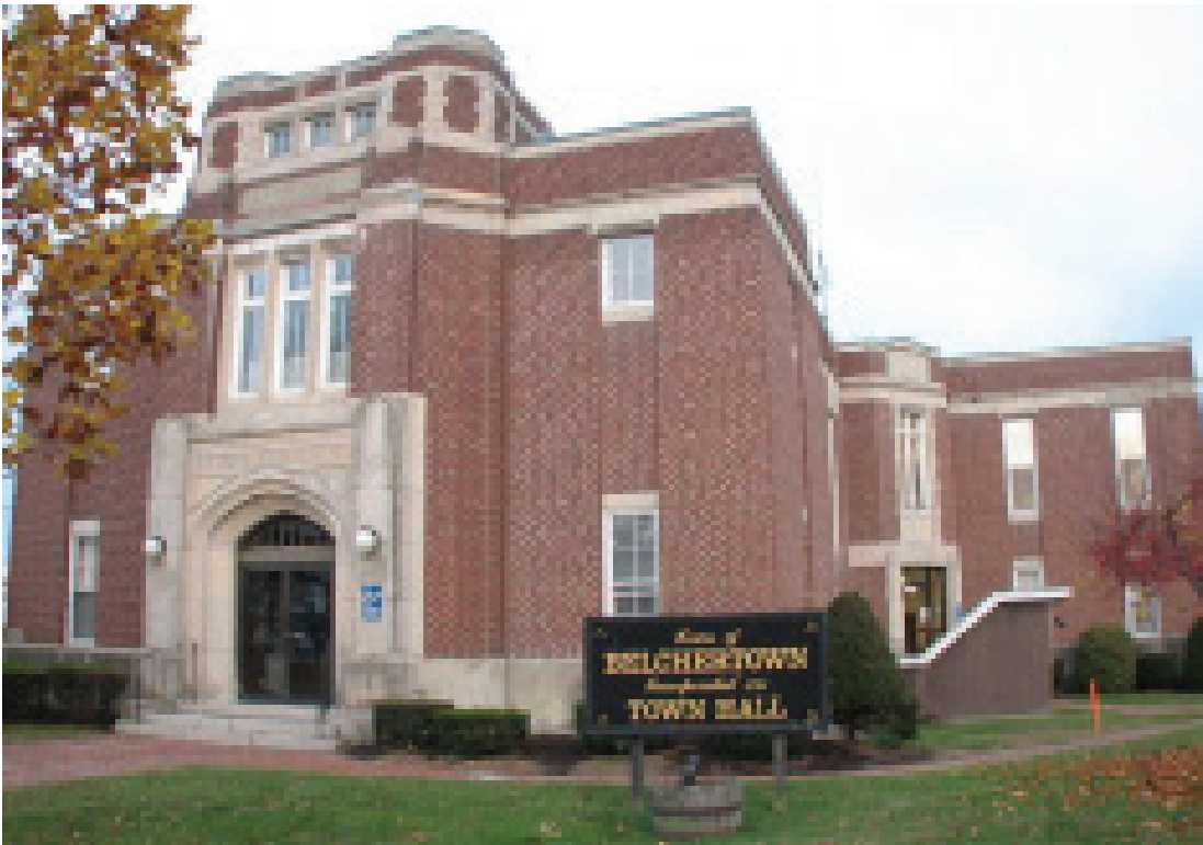
Belchertown Town Hall received energy efficiency upgrades in 2011
