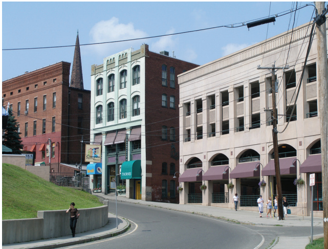
Northampton Parking Garage
