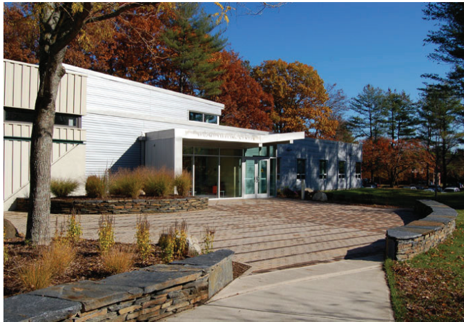
New 6,700 square foot addition to the Jerome Liebling Center for Film, Photography and Video, a part of the Arts Complex at Hampshire College.
