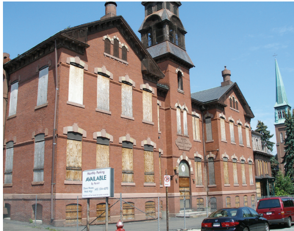
Former Holyoke Catholic High School
