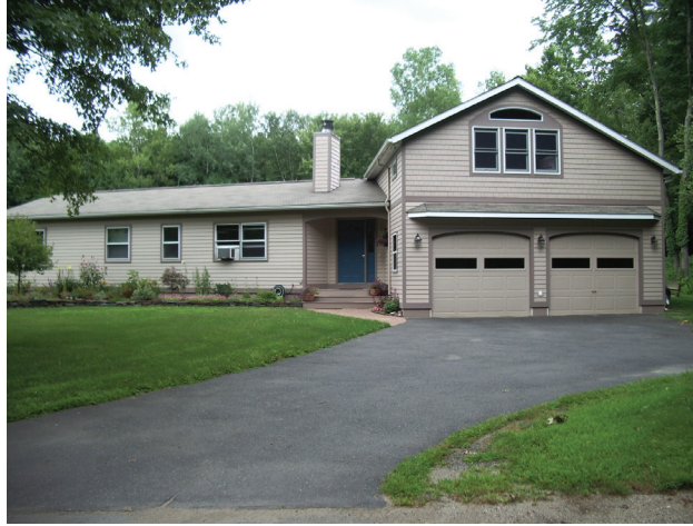
An accessory apartment over the garage in a single family house
