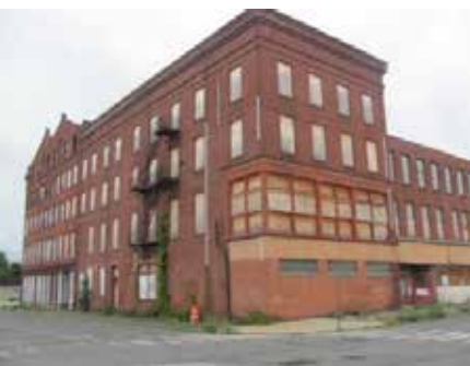
Silvio O. Conte corner - 345 Dwight Street, Holyoke. Located across from the future passenger rail platform in Depot Square, this vacant building originally had retail on the first floor with hotel/boarding rooms above. Source: City of Holyoke
