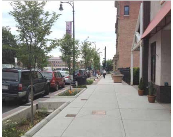
After: Street drains through curb cuts to bioretention planters.
