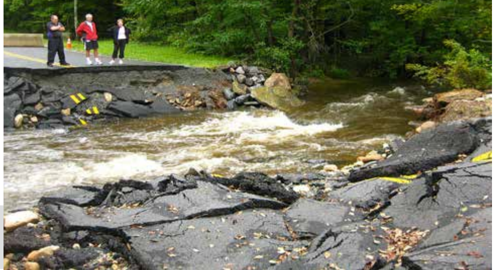
A key east-west Massachusetts highway corridor, Route 2, was washed out during Tropical Storm Irene.
