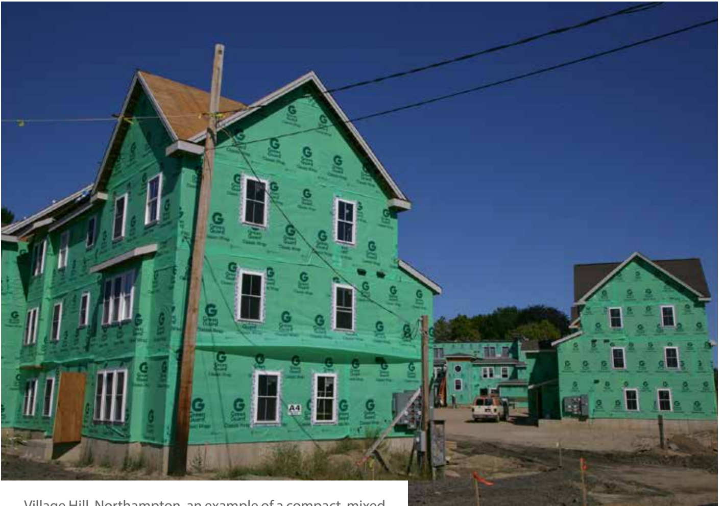
Village Hill, Northampton, an example of a compact, mixed-use energy efficient development
