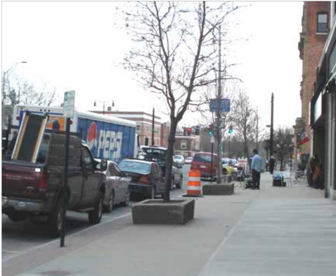
Before: Street drains to catch basins and storm drains
