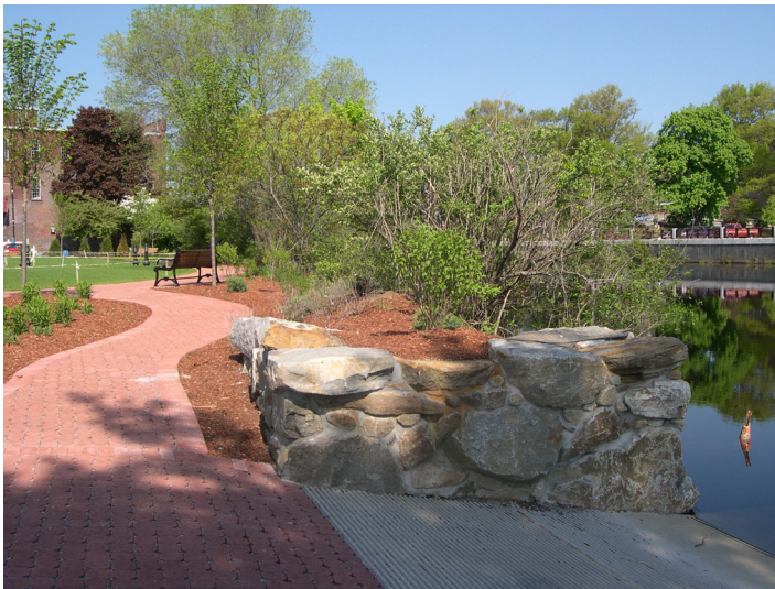
Pervious pavers used for the walkways at Riverfront Park in Orange, MA.
