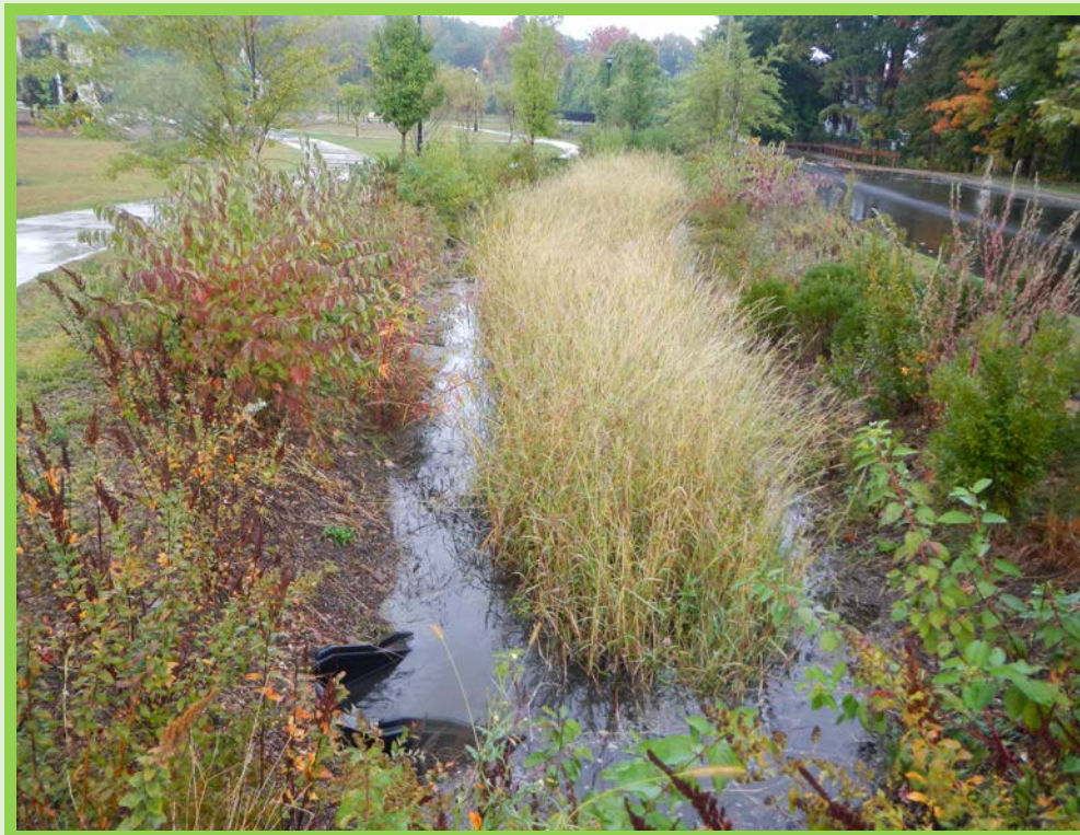
A bioretention basin helps to slow the flow at Community Field.
