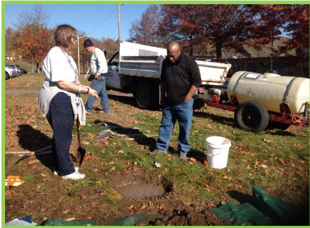
Holyoke Community College students wait for a percolation test hole to drain at Sullivan Elementary School. The City provided water for test holes with tank shown in background.
