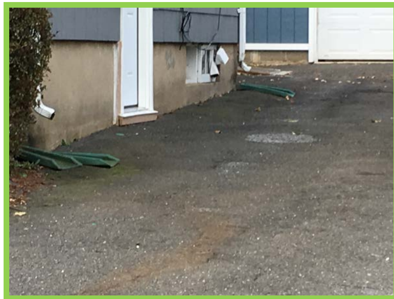
Rooftop flow from many neighborhood homes spill to driveways that then deliver flow to roadways and street drains/catch basins that tie to the Day Brook pipe.
