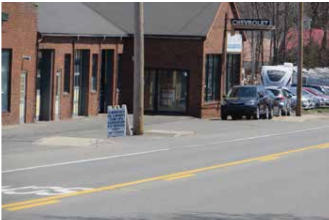
Sidewalk on the north side of Route 9 looking east toward Haydenville
