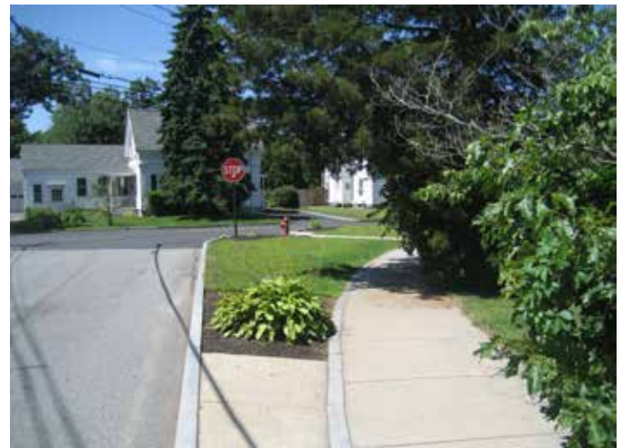
(B) Grass, trees and extended sidewalk in curb extension
