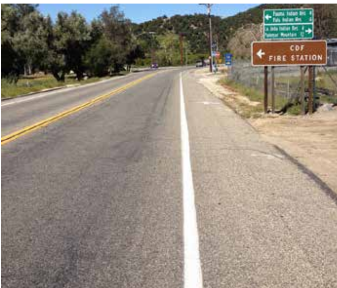
Fog lines delineate the vehicular driving zone on wide roadways.
