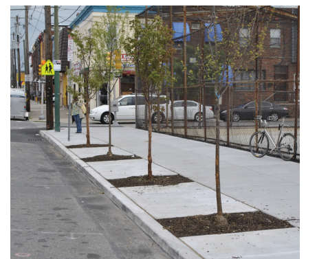
Example of an easily maintained covered tree trench on Washington Avenue in Philadelphia, PA
