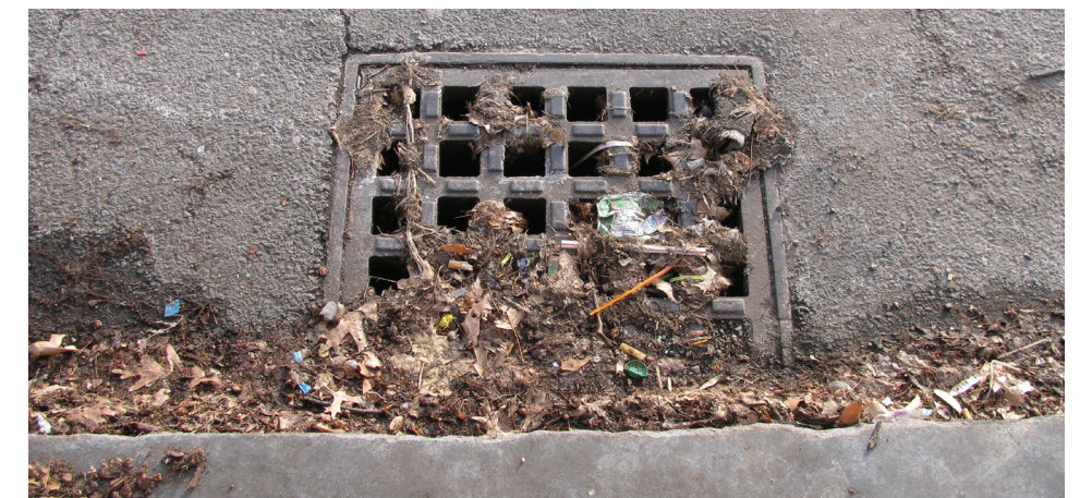
Inlet on Belmont Avenue
