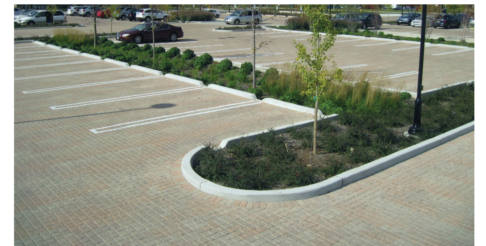
An permeable parking lot with infiltration planters in Carol Stream, IL
