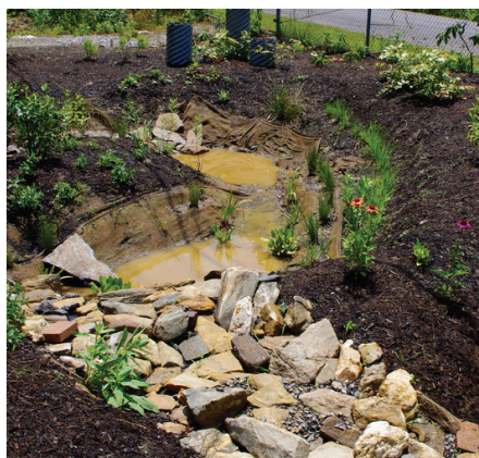
A channel that catches water and directs it to the raingarden.
