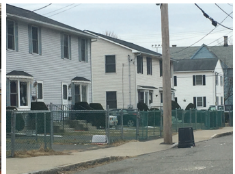
Center Street is lined with fenced in duplex housing with a sprinkling of historic, brick buildings.
