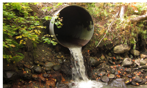
A CSO outlet empties into a stream
