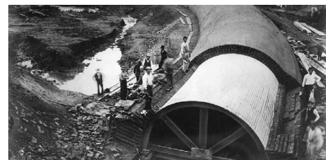
A CSO system being constructed in Philadelphia in 1883
