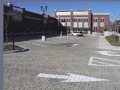
Elmwood Ave. Largest permeable parking lot in New England
