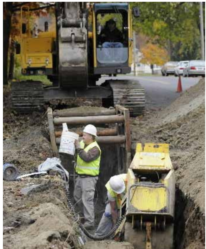
Stormwater sewer separation project from 2012 in Chicopee.
