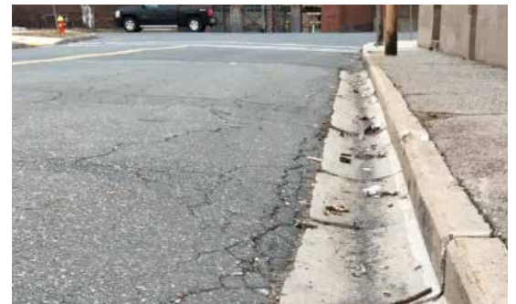
Runoff is directed along the curbs, carrying debris with it on its way toward catch basins along the road.
