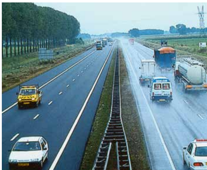
Visible differences in surface water with pervious asphalt (left) and regular asphalt (right) on a highway in the Netherlands.
