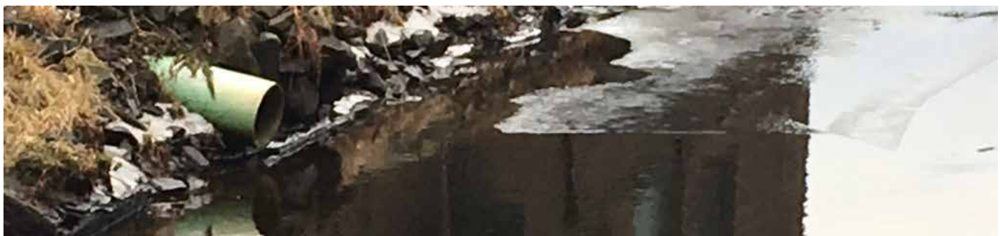
A main stormwater outfall from downtown Chicopee to the Cabotville Mill canal. Photograph by the authors.
