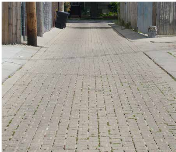
Permeable pavers in the form of bricks. Consistent spacing filled with sand allows water to infiltrate.
