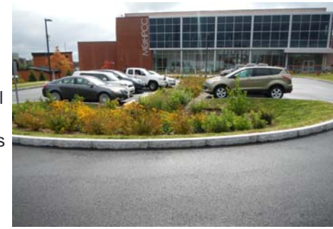
Massachusetts Green High Performance Computing Center, Holyoke
