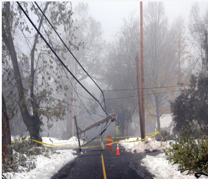
Above ground electrical infrastructure is vulnerable to damage from heavy winds and freezing precipitation.
