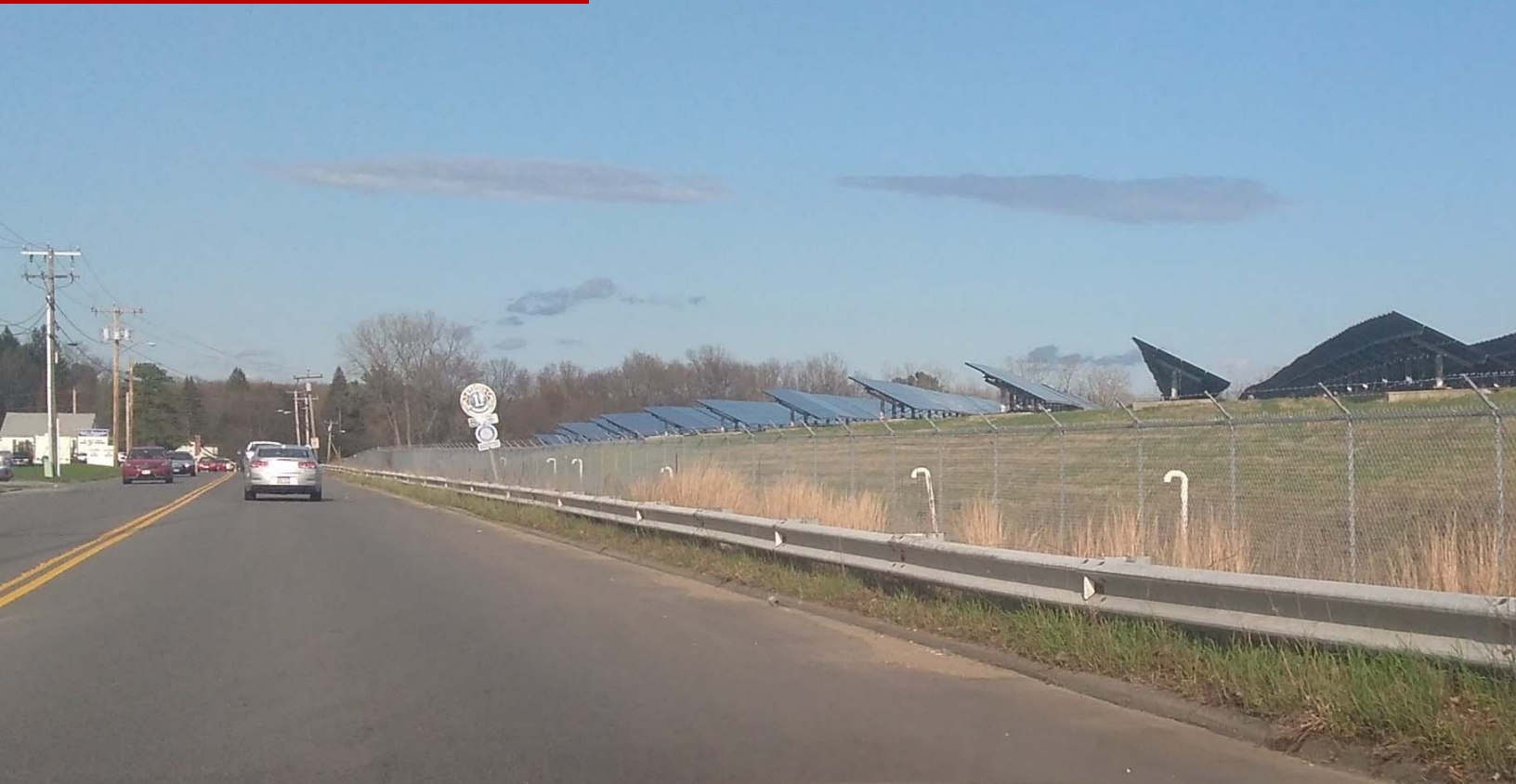
Photo: Solar Farm off Holyoke Street in Ludlow, MA
