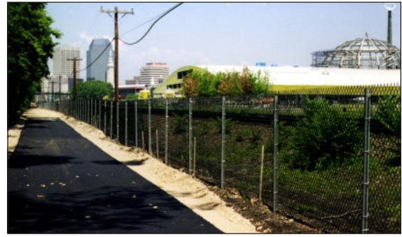
Connecticut RiverWalk and Basketball Hall of Fame under construction
