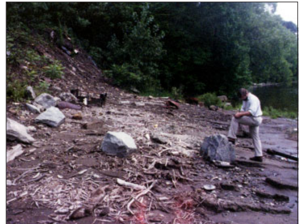
Chicopee CSO outfall
