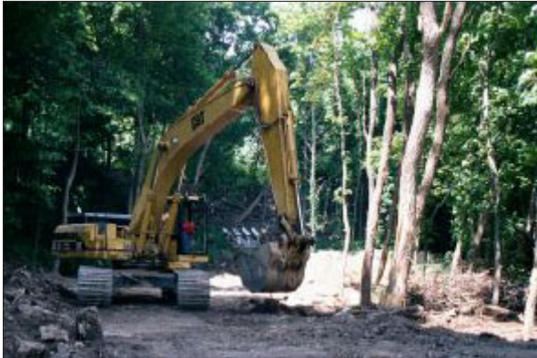
Holyoke sewer separation
