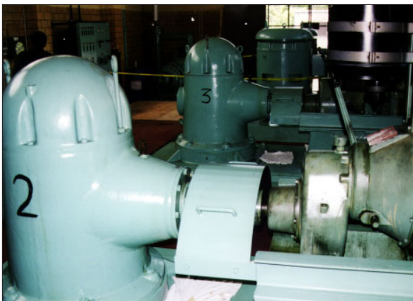
Pump rehabilitation at Springfield's York Street Pump-Station
