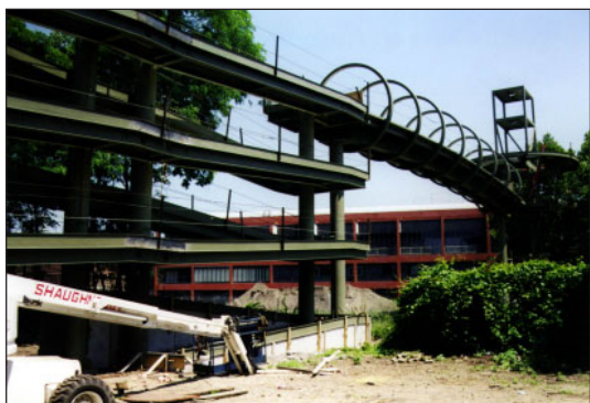
Connecticut River Walk construction
