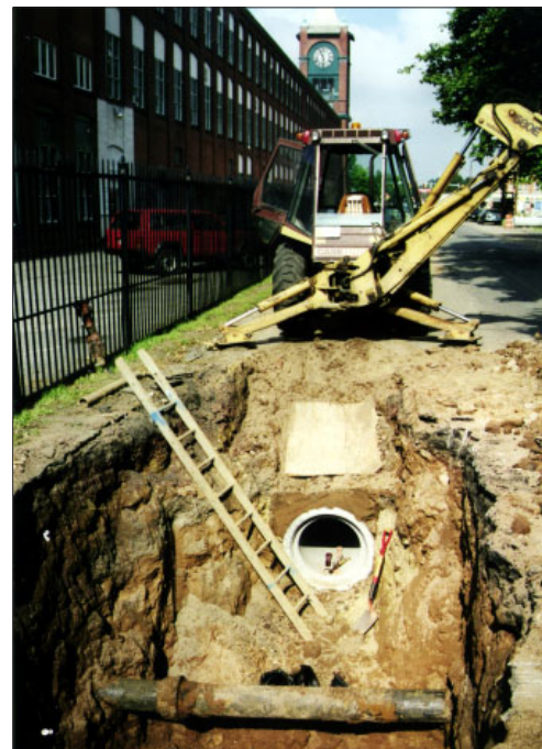
Ludlow sewer separation
