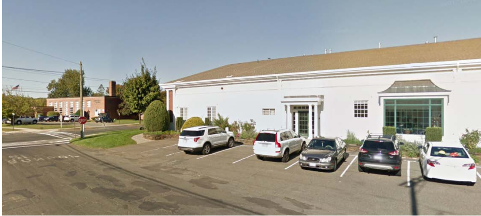
Location: Cold Spring Avenue/Baldwin Avenue, Memorial School on left Description: lack of controlled access and no off-street parking aisle.
