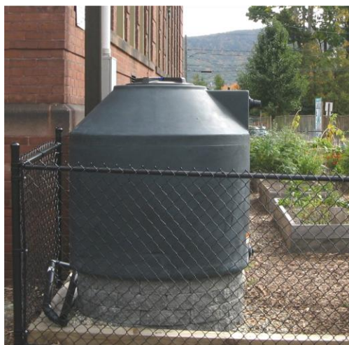
Cistern - Center Pepin Elementary School, Easthampton
