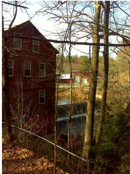
Lyman's Mill and Dam at Mill Pond
