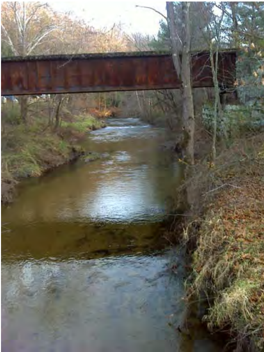
Bridge Crossing at Gunn Road
