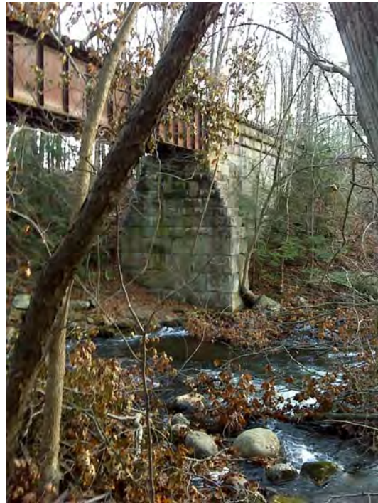
Bridge Crossing at Mill Pond
