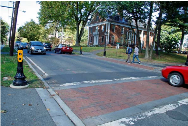
Raised Intersection, College Street, Amherst
