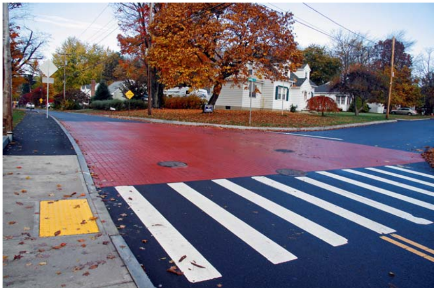
Textured Pavement at a Raised Intersection on Grove Street, Northampton causes cars to slow down through visual cues and textural changes
