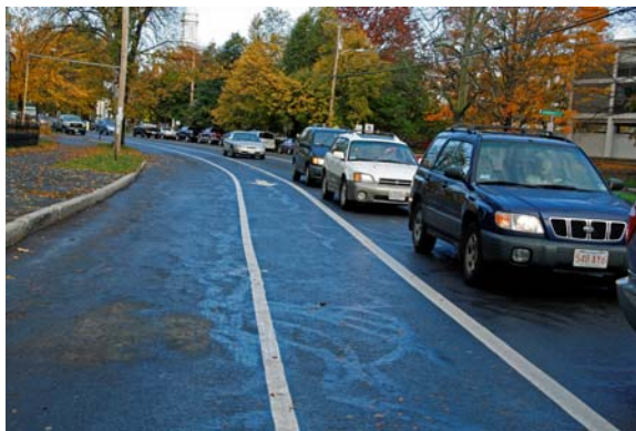
Road Narrowing on Elm St, Northampton: Painted lines and bike lane are used to narrow the auto lane
