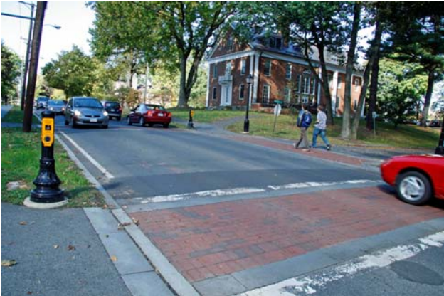
Raised Intersection, College Street, Amherst
