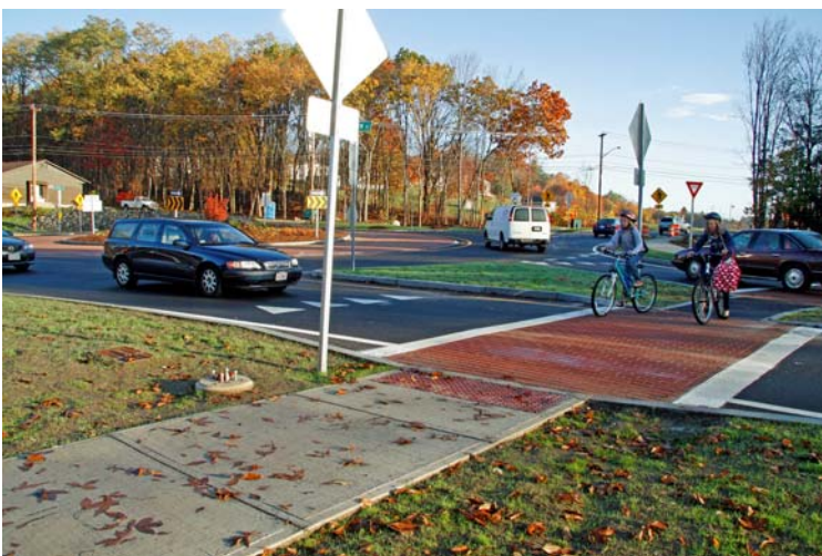
Splitter island provides a resting area and narrows lane widths at crossing points
