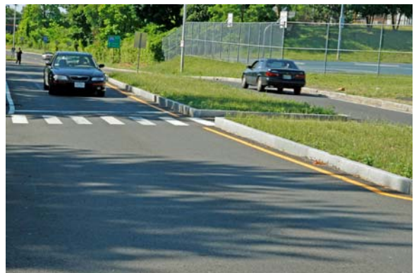
Resnic Boulevard pedestrian refuges are fitted with a gap along the crosswalk
