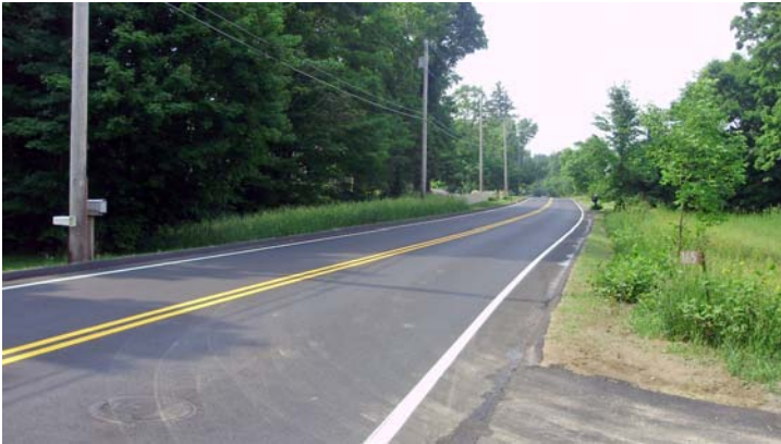
New pavement markings establish narrower 10 foot travel lanes on West Farms Road, Northampton
