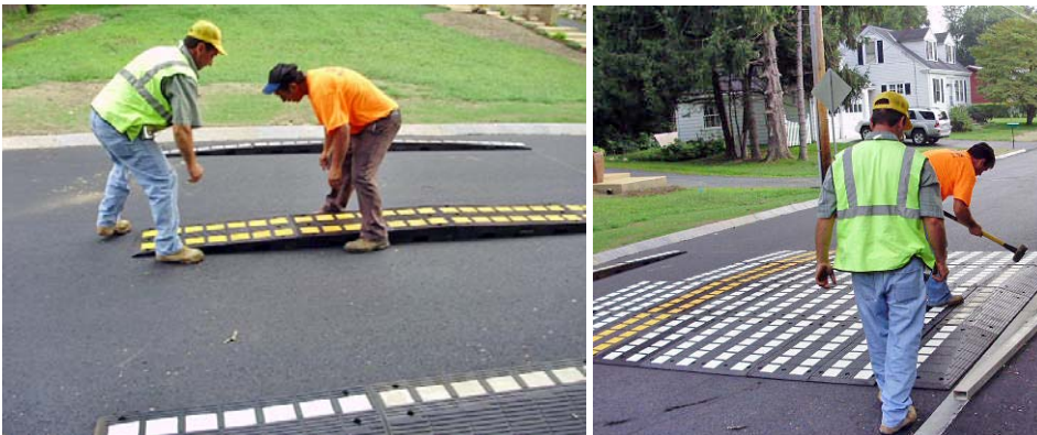
Installation of a permanent speed hump on Grove Street, Northampton
