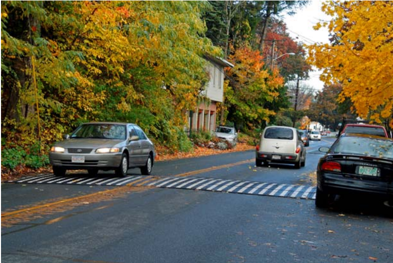
Temporary Speed Hump, State Street, Northampton
