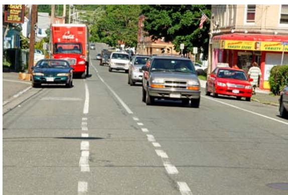
Dwight Street: One travel lane, two parking lanes, and a bike lane
