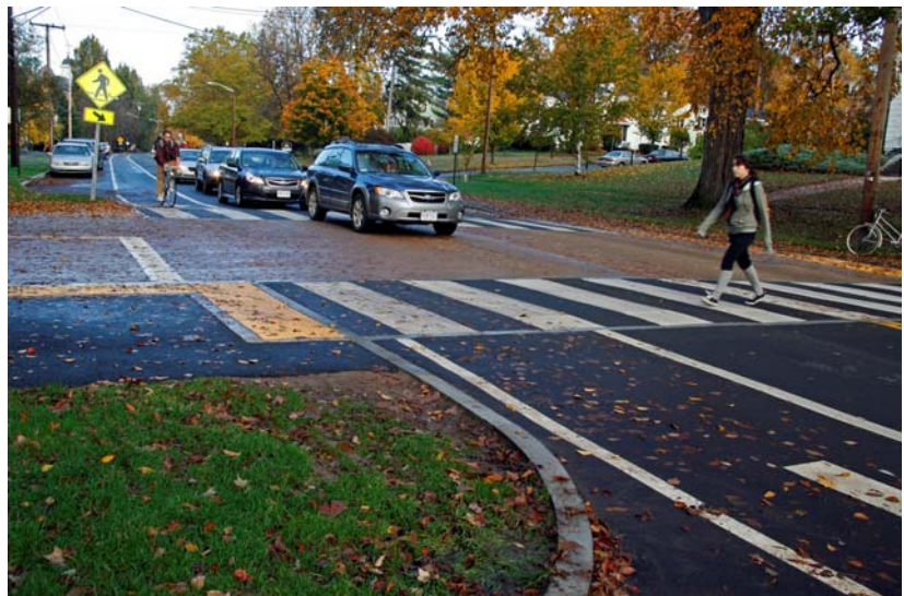
Raised Crosswalk, Elm Street, Northampton
