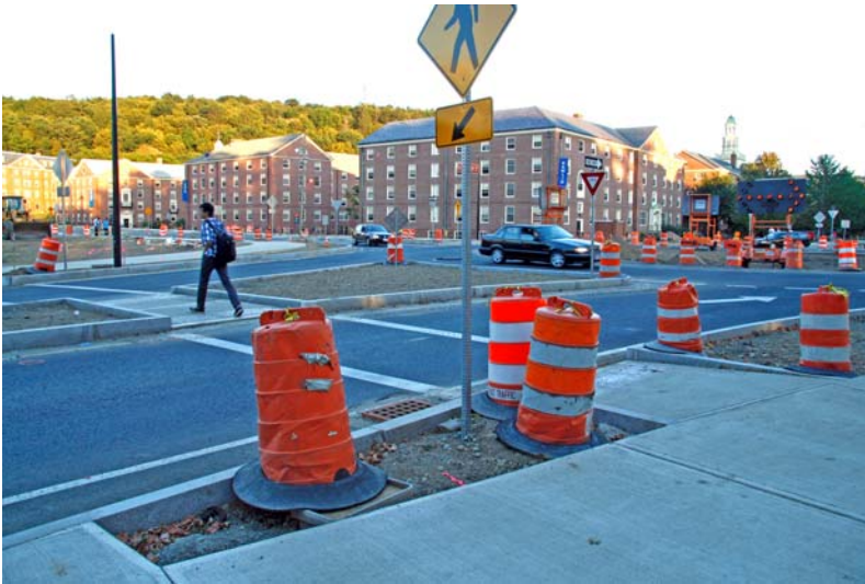
Modern Roundabout under construction at UMass-Amherst
