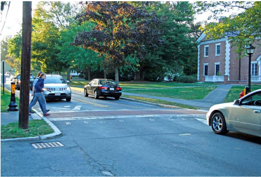
Raised Crosswalk in Amherst. Bollard light flashes when crossing (left)
