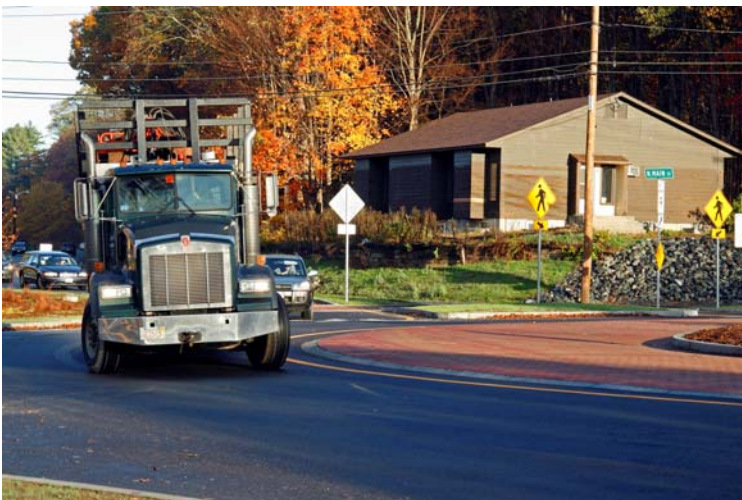
Brick pavement at center creates a narrow travel lane and allows extra room for large turning radius vehicles
