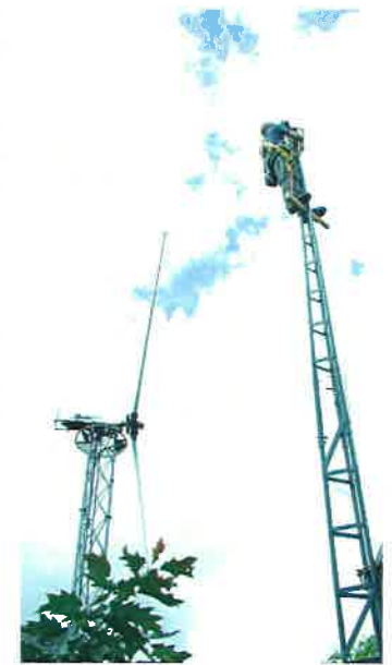
Solar Sensor Installation - Mt. Tom, MA
