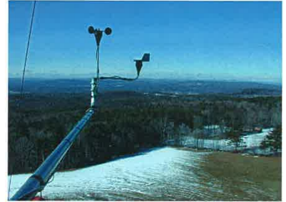
Anemometry Installation - Northfield, MA
