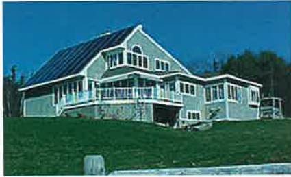
This solar home, constructed by Maine Solar House, generated 2,051 kW hrs of electricity from its integrated roof array in 6 months.
