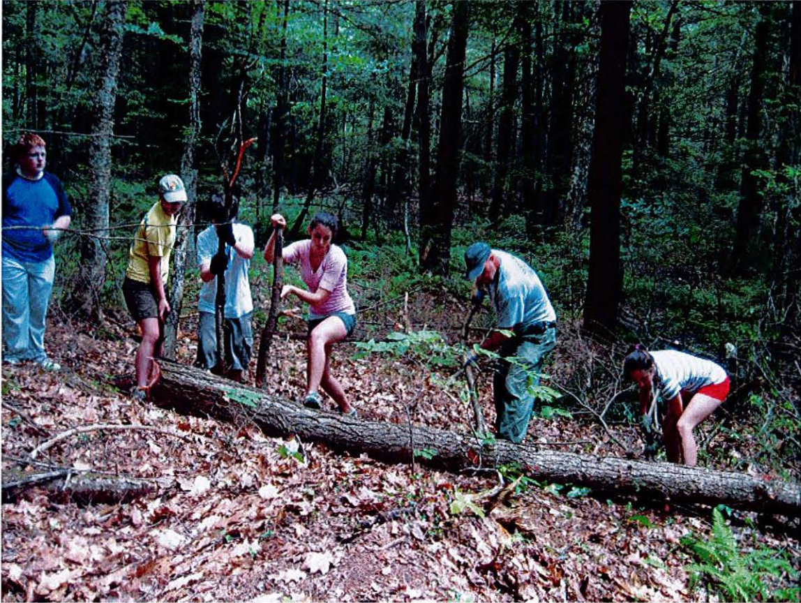
Tilton Farm trail construction crew, June 2010
