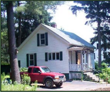
FIGURE 16: Before photo, home on Warren, MA. Dilapidated front porch, front façade, and roof.
