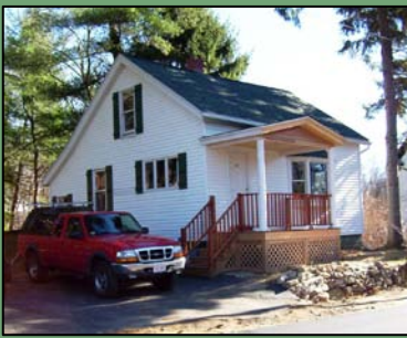
FIGURE 17: AFTER PHOTO. NEW PORCH, NEW FRONT FAÇADE AND NEW ROOF.
