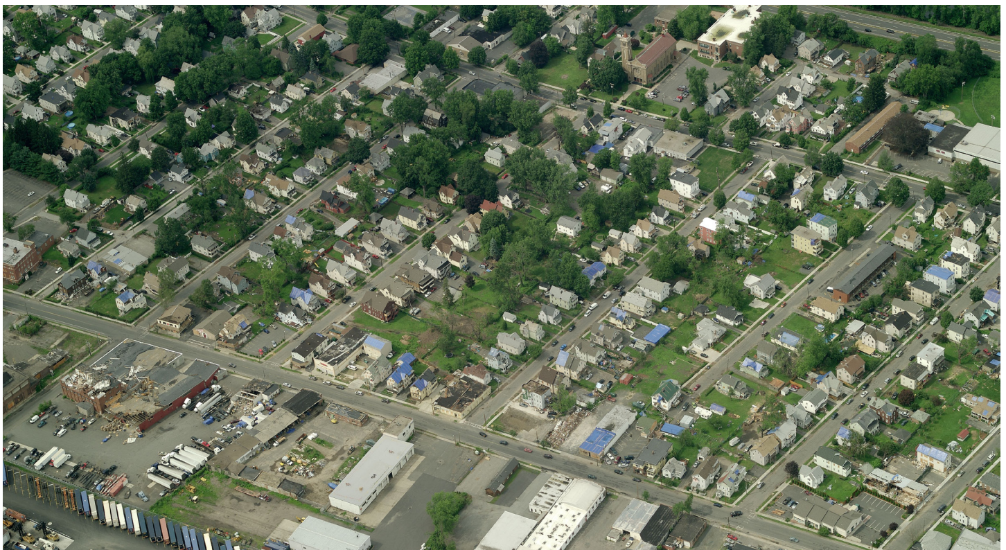
Southern Section of Merrick after the June 2011 Tornado. Blue tarps cover damaged roofs and the tree canopy was decimated in the tornado's path. Image courtesy of Pictometry International – Rochester, NY. Copyright 2011.
